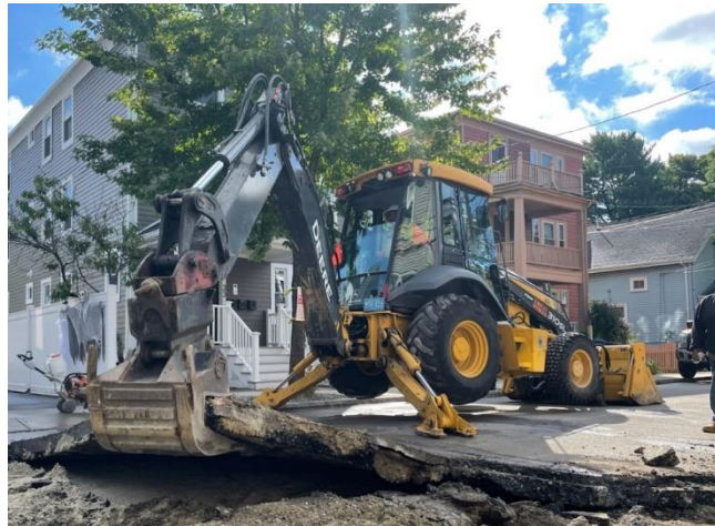
Repairing a street
