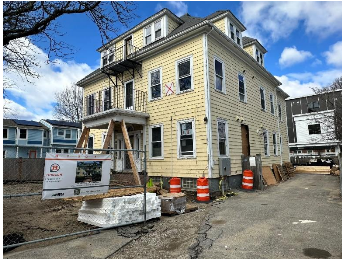
Renovations underway at 35 Harvey Street
