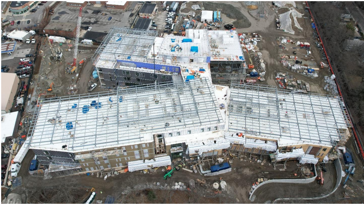
Construction of the Tobin Montessori & Vassal Lane School
