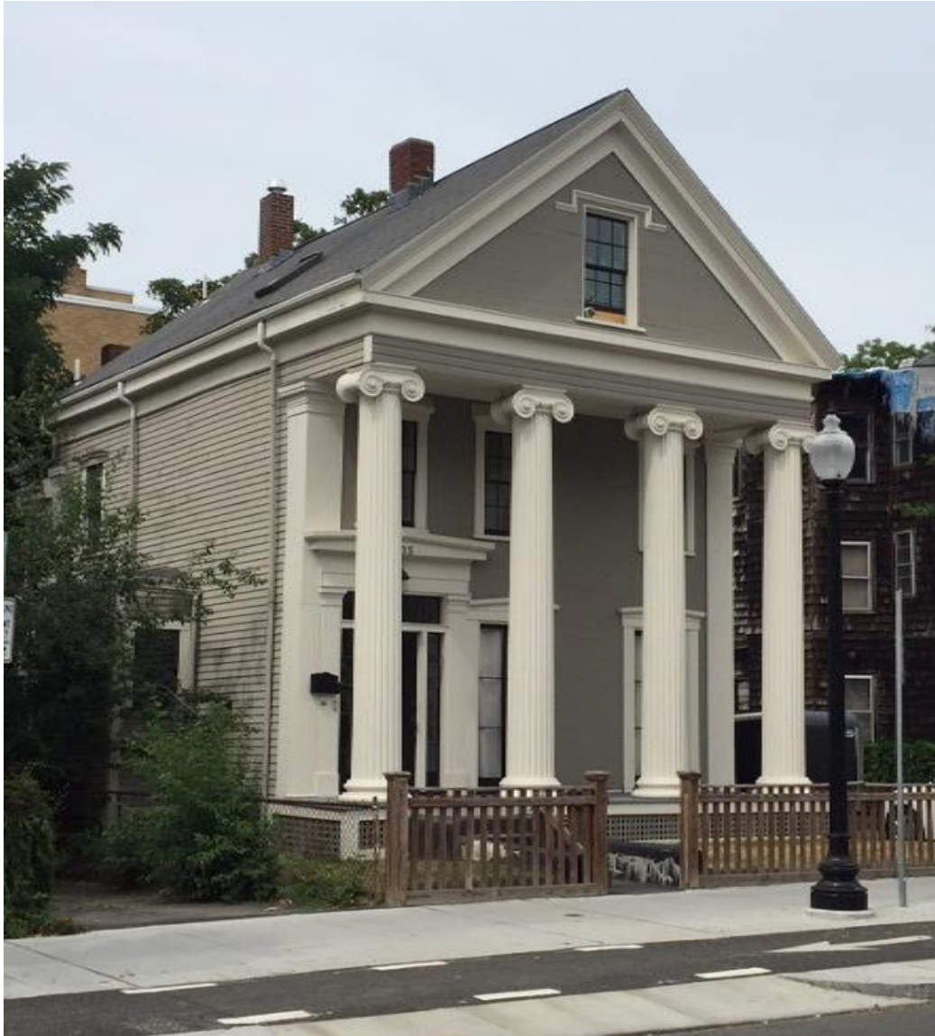
135 Western Avenue, July 28, 2016
