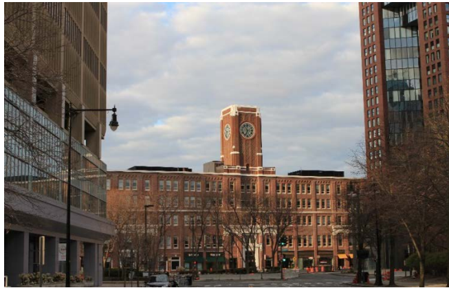
Existing view looking down Third St toward Main St
