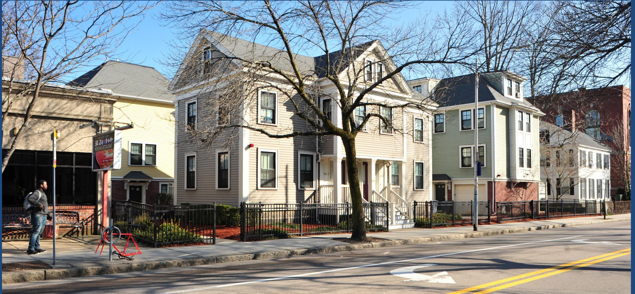
PG 20-04, 156 Prospect Street, by Just A Start. $40,000 for exterior trim repairs
