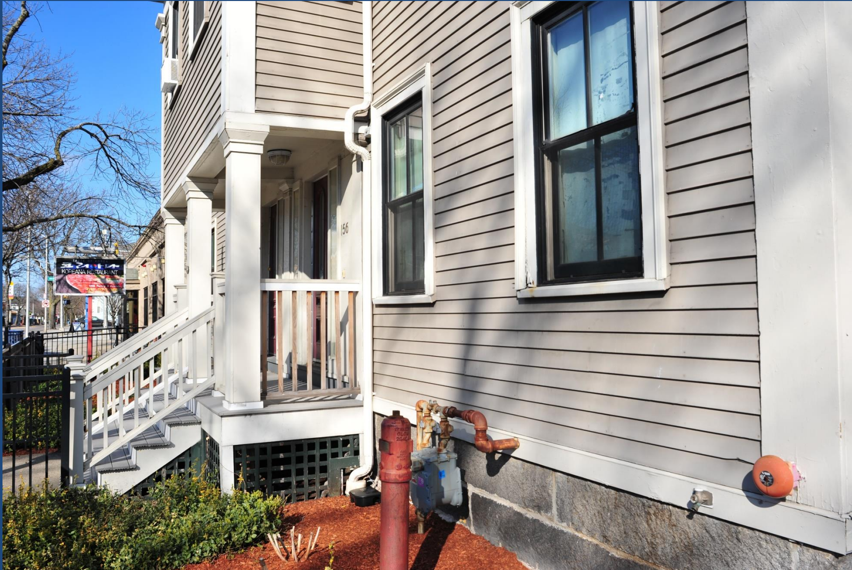
PG 20-04, 156 Prospect Street, by Just A Start. $40,000 for exterior trim repairs
