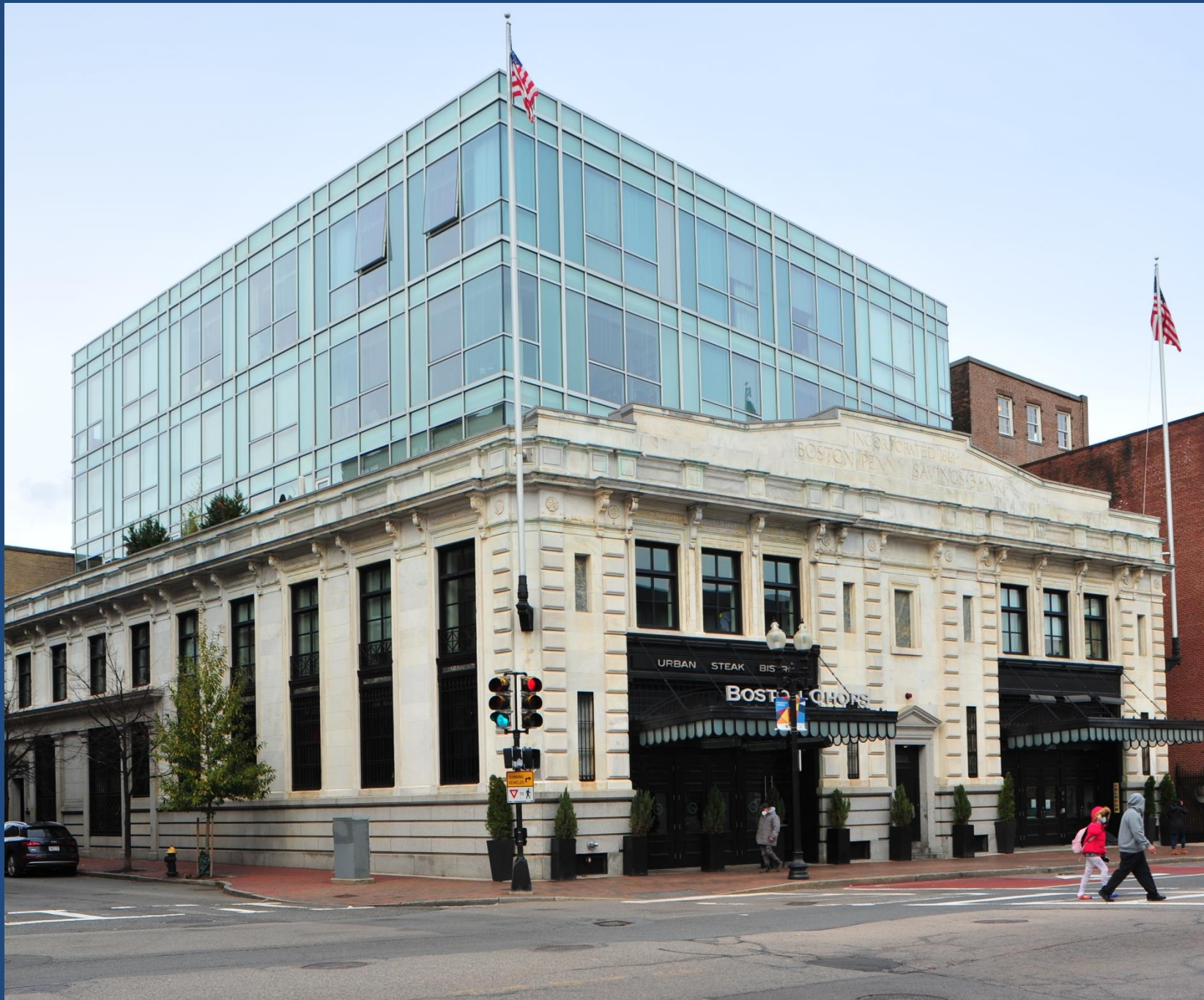
Boston Penny Savings Bank, 1367 Washington St., Boston Finegold Alexander Architects (2007)
