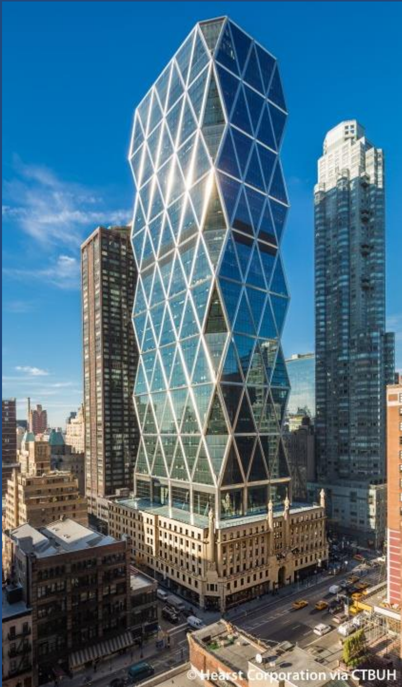
Hearst Tower (1928, 2004) 300 W. 57 th Street, NYC Norman Foster, architect
