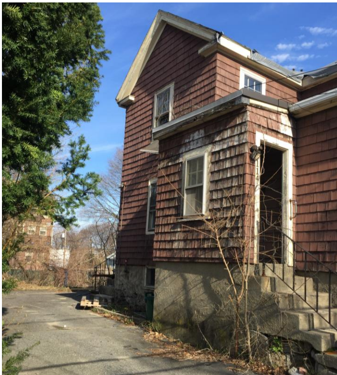
114 Clay Street, CHC photo, 2018
