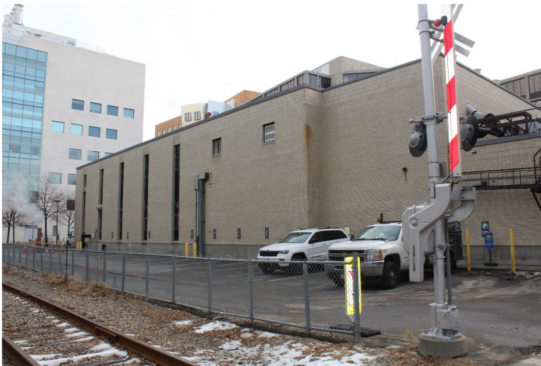
51 Vassar Street, MIT Building 44, rear elevation. CHC staff photo, 12/26/19
