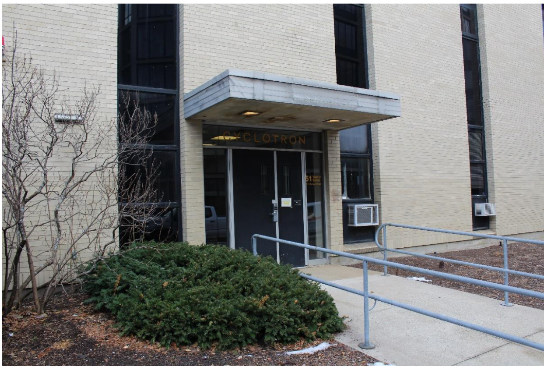
51 Vassar Street, MIT Building 44, Vassar Street entrance. CHC staff photo, 12/26/19
