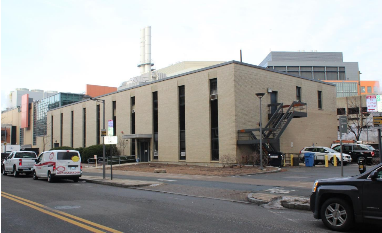
51 Vassar Street, MIT Building 44, facing west on Vassar Street.
