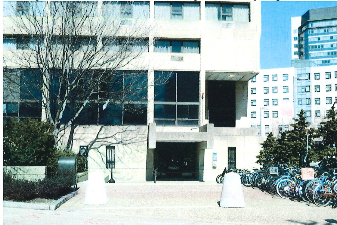
Entrance on west elevation, looking east from Wadsworth Street.
