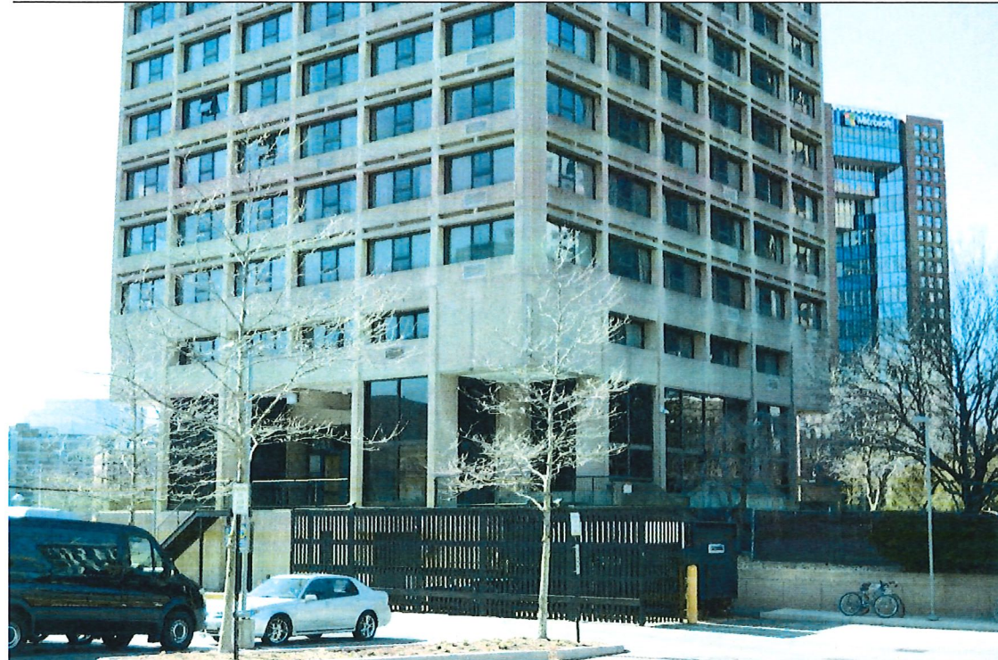
Detail of ground level, south and east elevations, looking northwest from parking lot.
