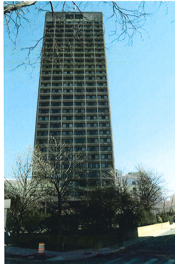
North elevation, looking south from opposite corner of Wadsworth and Main streets.
