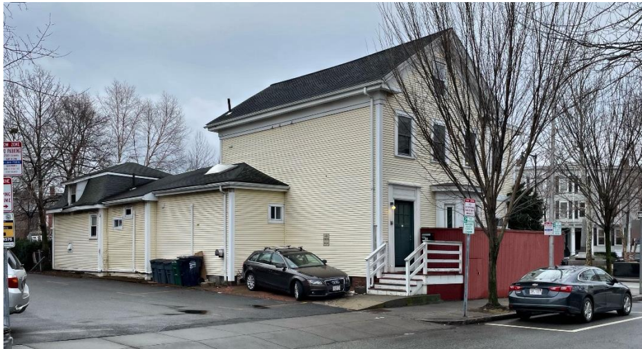
18 Pleasant Street, northeast side facade.
