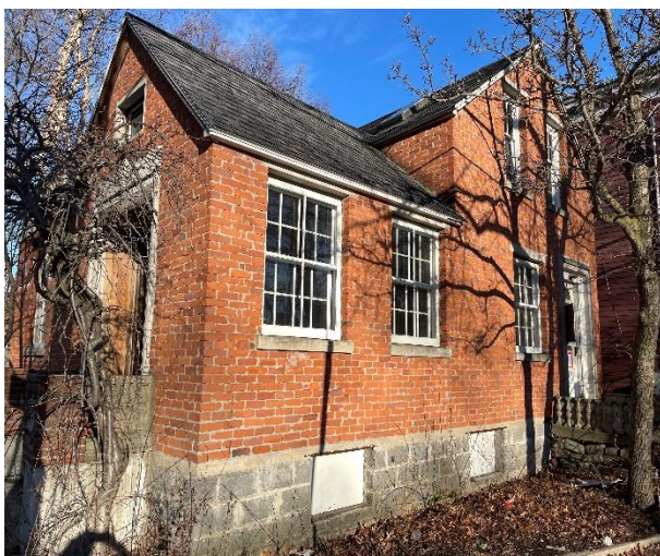
235 Third Street façade.
