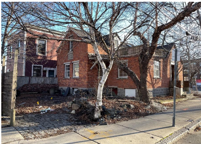
235 Third Street, west and south facades from Bent Street.
