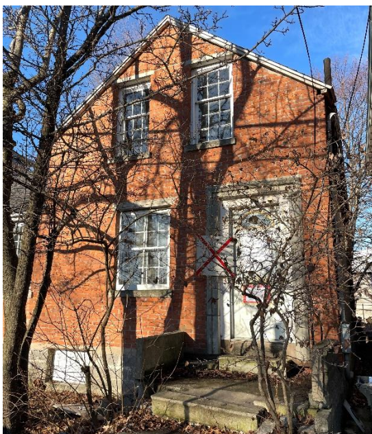
235 Third Street façade.
