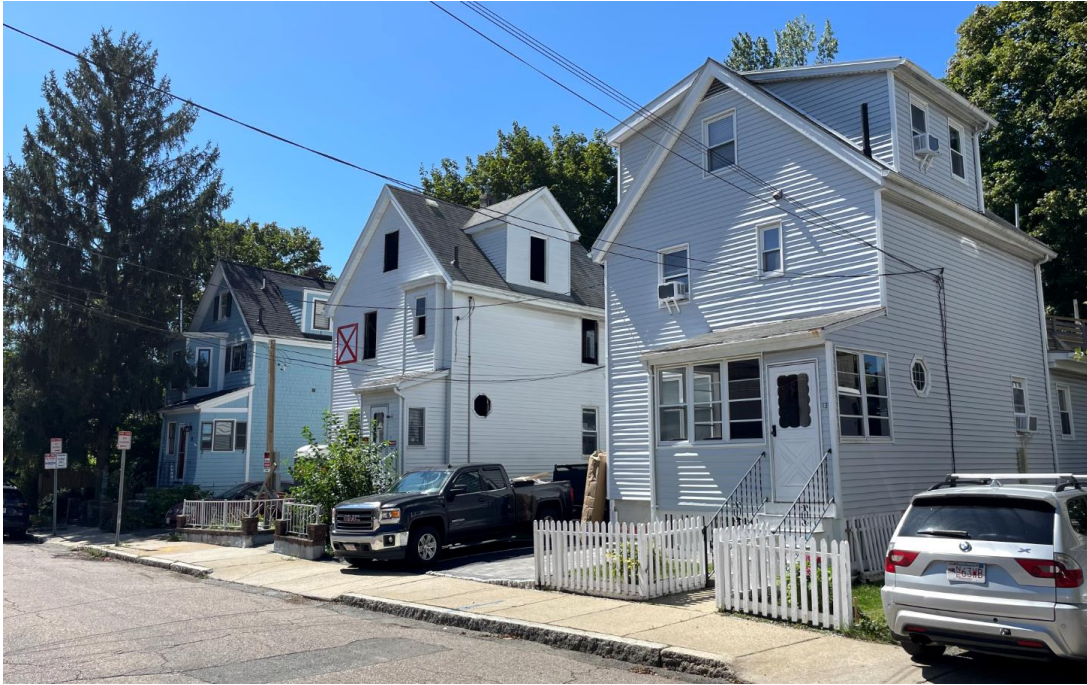
From right to left: #13, #19, and #21 Cottage Park Avenue. All similar in overall design with varied later alterations.
