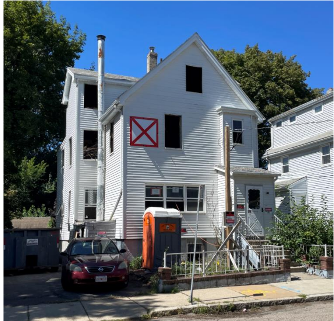
19 Cottage Park Avenue, CHC Photo, 09-01-2023
