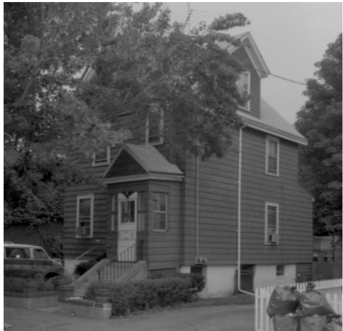
19 Cottage Park Avenue, CHC Photo, 1982.
