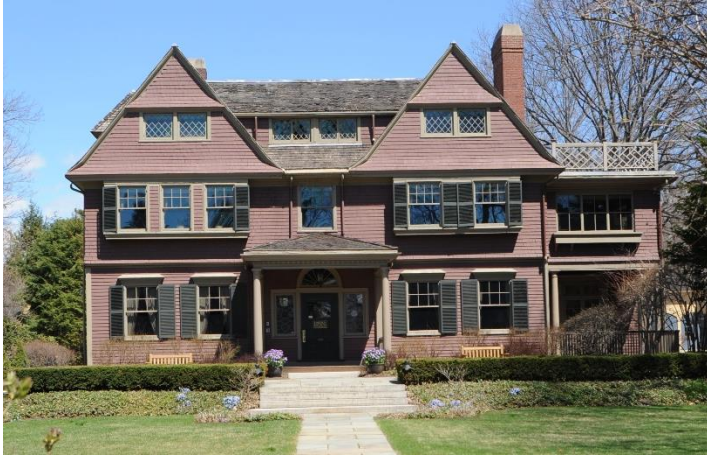
113 Brattle St. (1887, Andrews, Jaques & Rantoul, architects)
