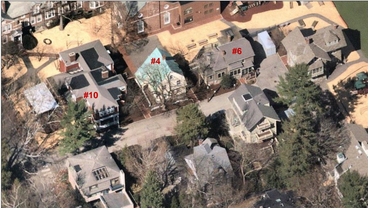
Aerial view of Buckingham Place, 27 March 2021. Nearmap.com accessed 5 Nov. 2021.
