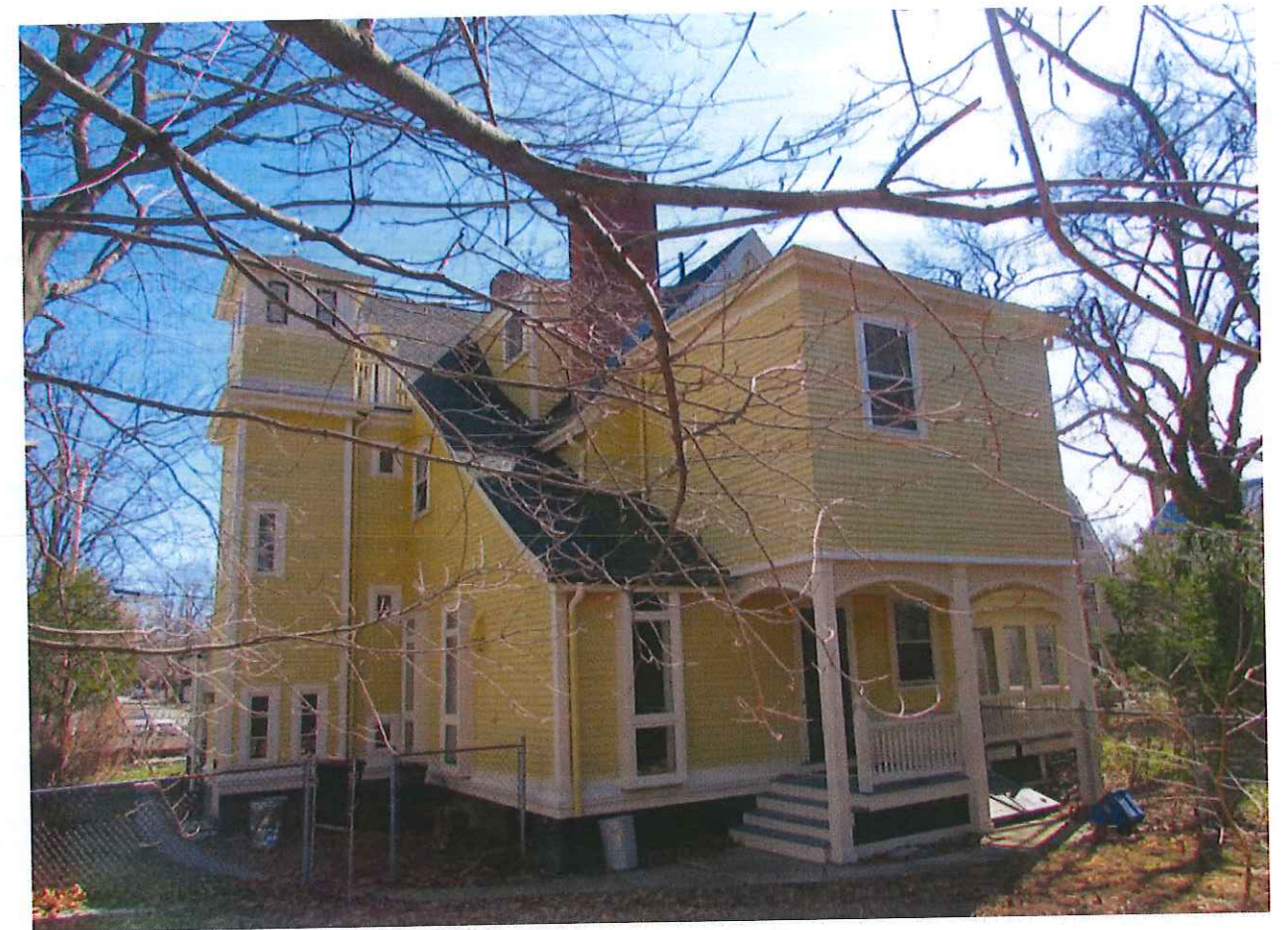
Existing North/West Elevation taken on property
