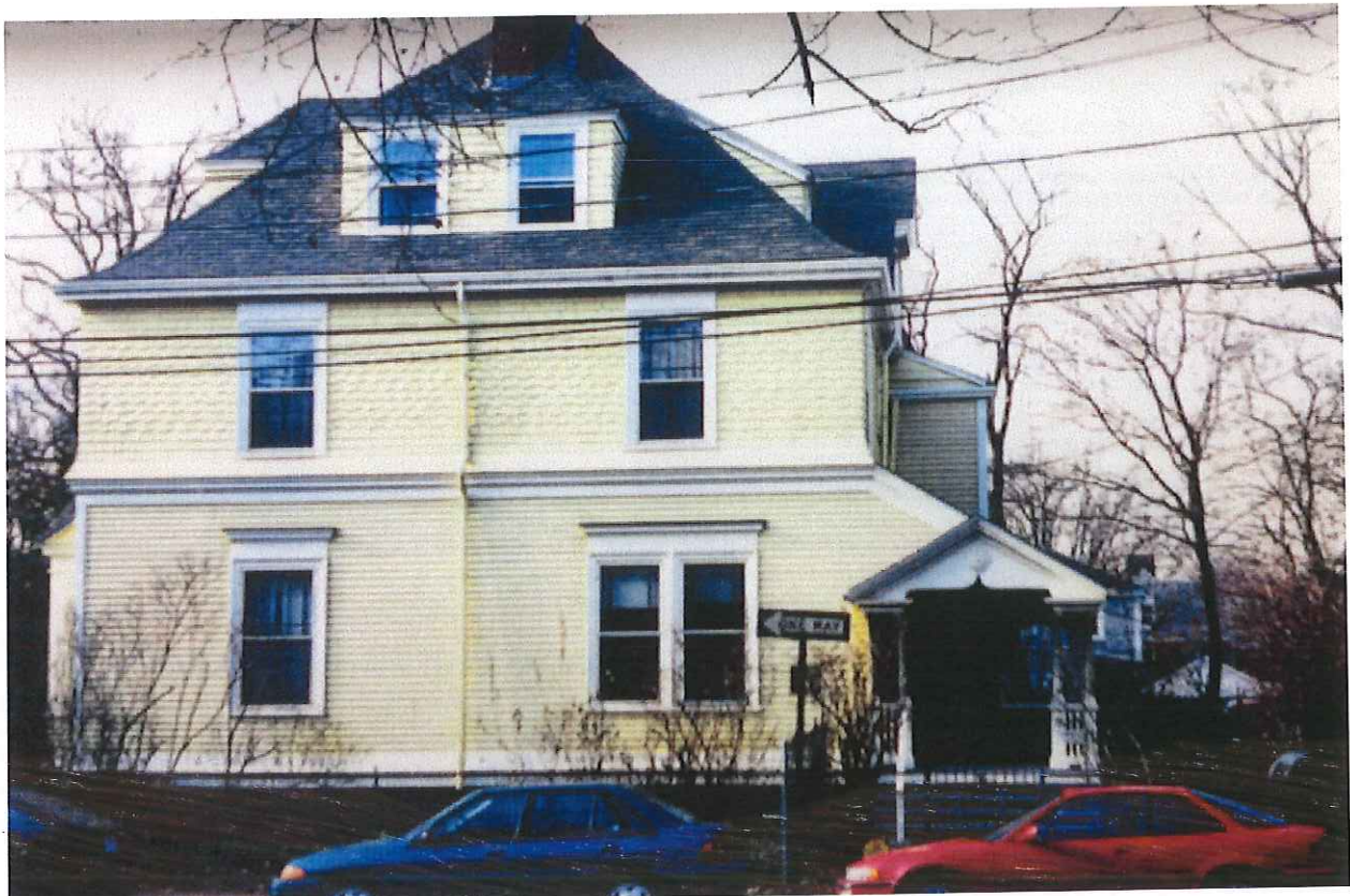
1996 Image Image from Building Department Files
