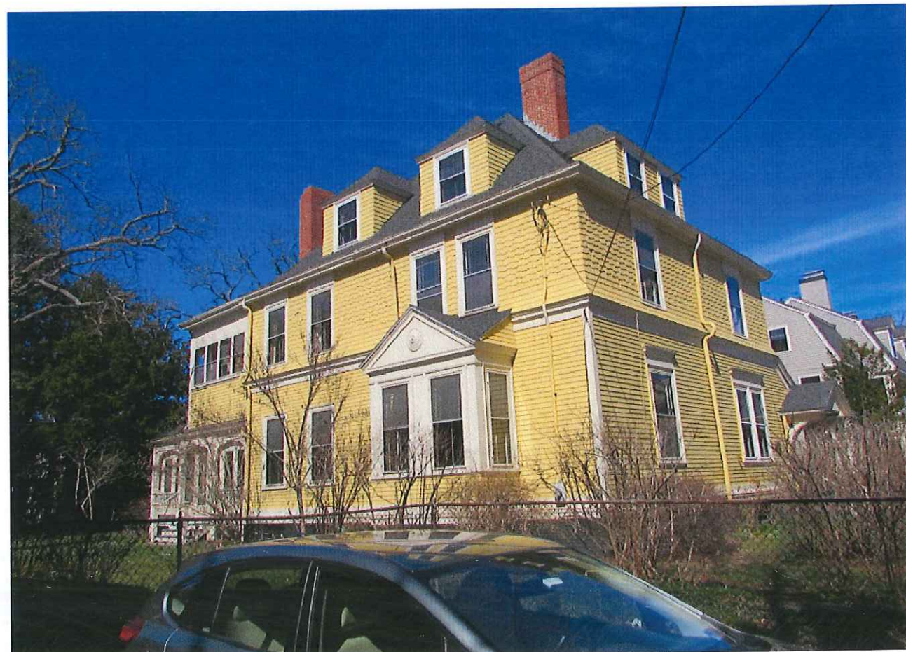
Existing South Elevation taken from Hawthorn Street 03.13.2016
