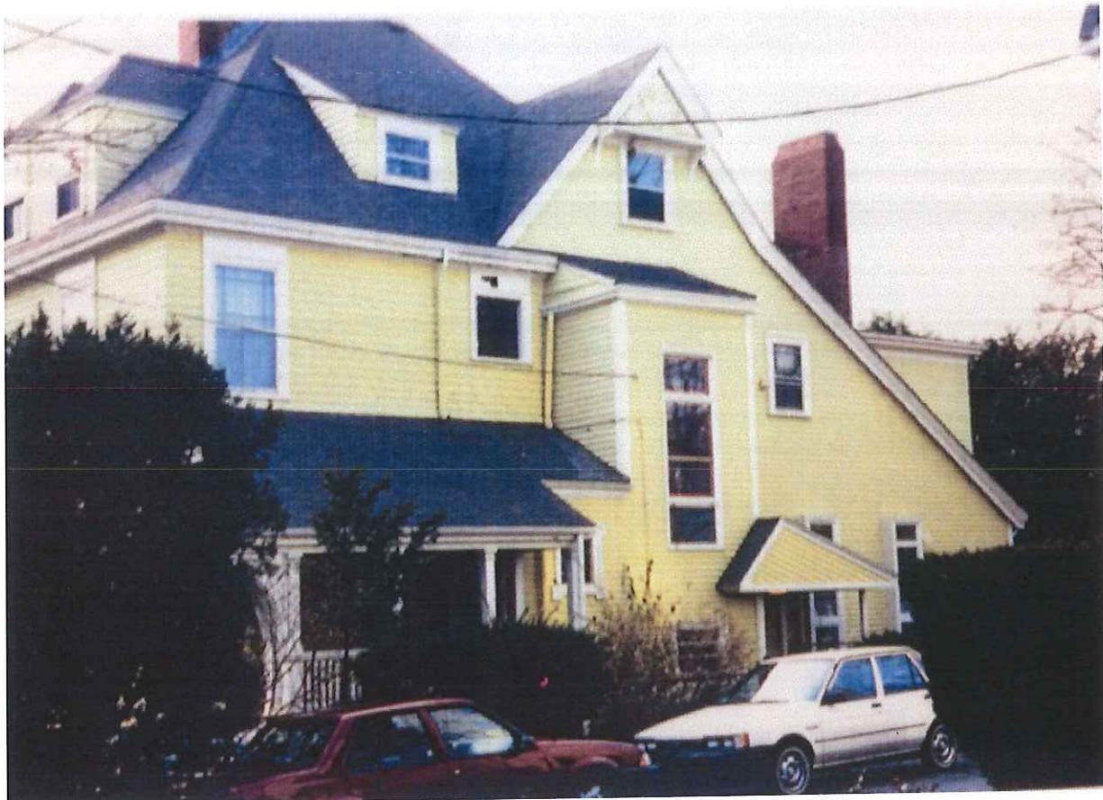
1996 Image Image from Building Department Files
