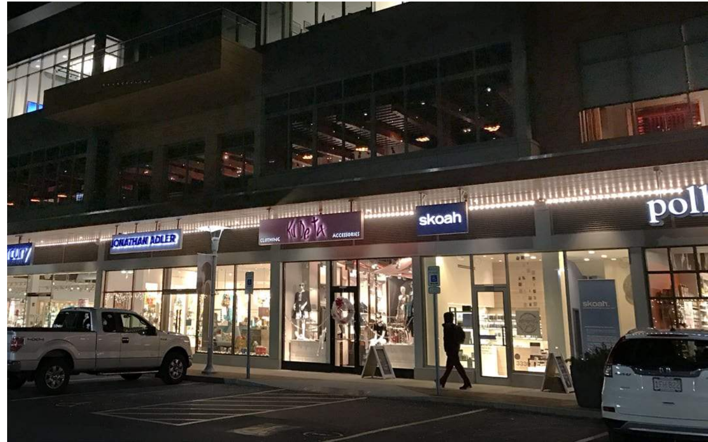
THE STREET, CHESTNUT HILL (ground floor retail, 2nd floor restaurant, 3rd floor office)
