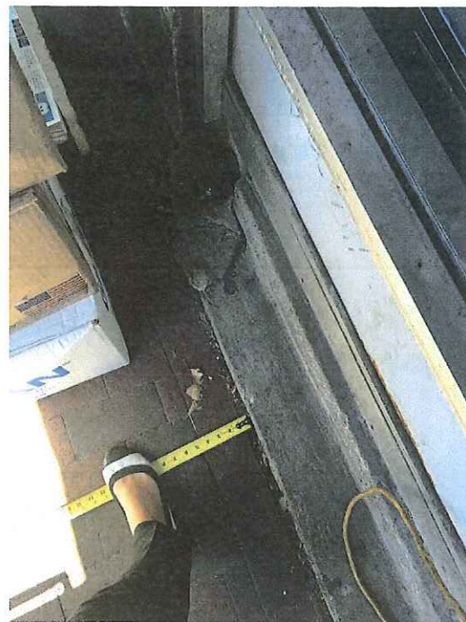
CLOSE UP OF BRICK AND CURB CONDITIONS
