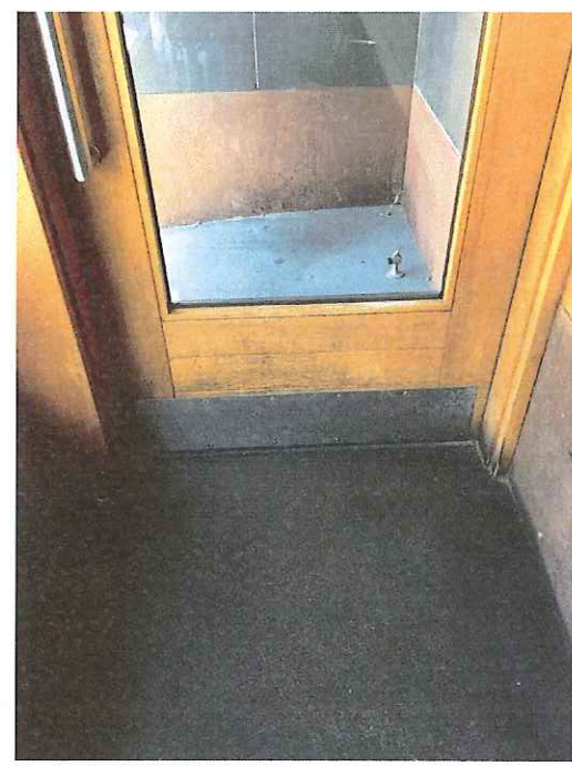
EXISTING CONDITIONS OF PROPOSED SECONDARY EXIT
