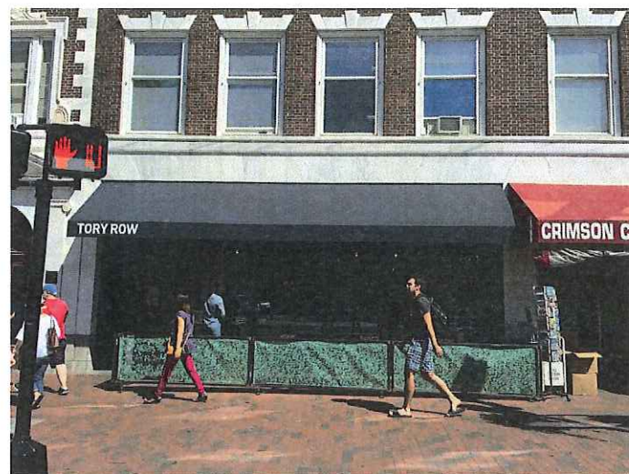
EXISTING TORY ROW FACADE AND PATIO CONDITIONS
