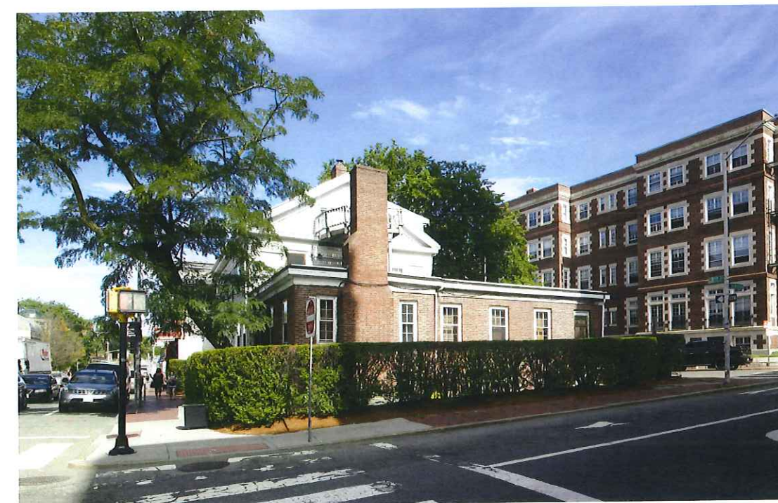
2 Looking at East Elevation from Mt. Auburn St. Scale: N/A
