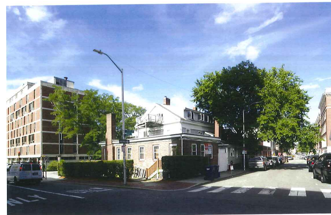
3 Looking at East Elevation from Bow Street Scale: N/A
