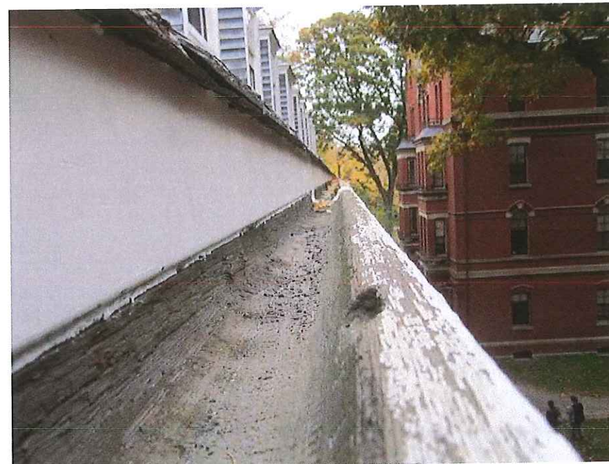
Interior of wood gutter
