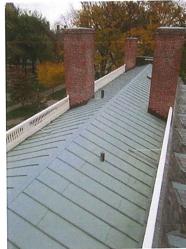
Standing seam copper roof and chimneys
