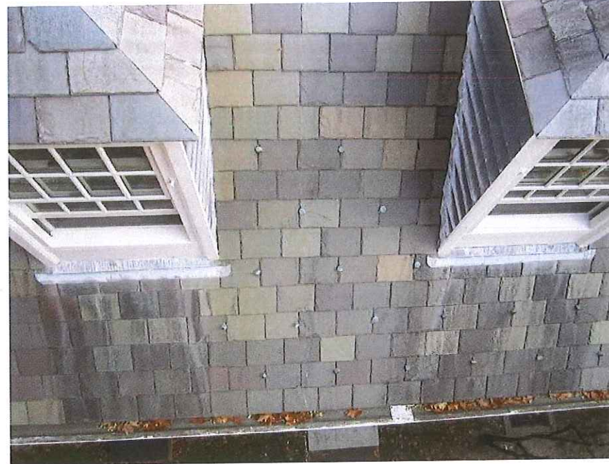
Slate roof detail showing existing snow guards at south elevation
