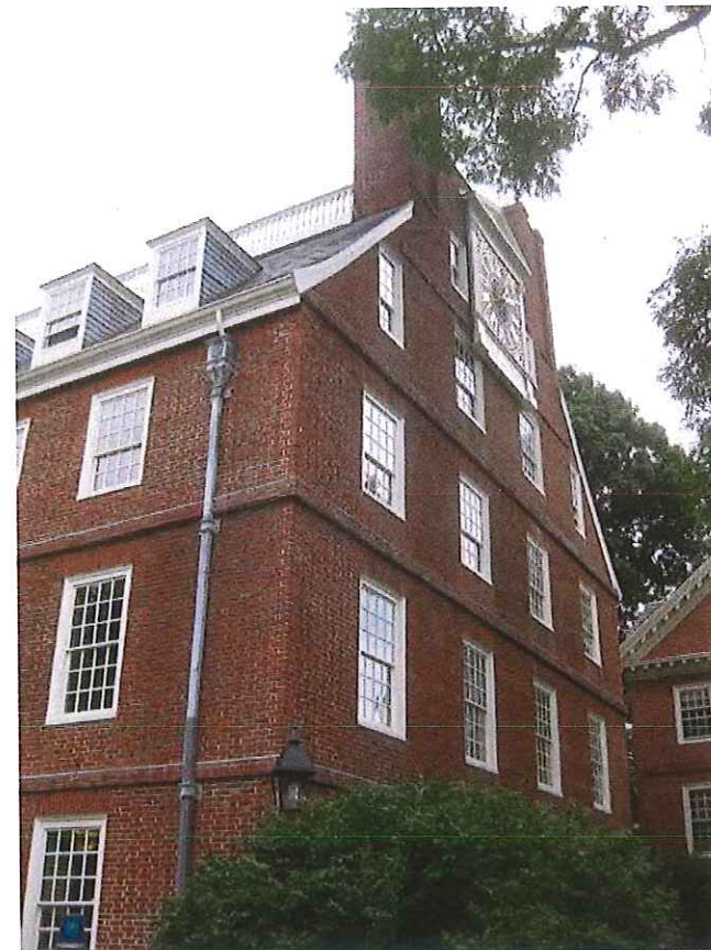
West Facade with clock
