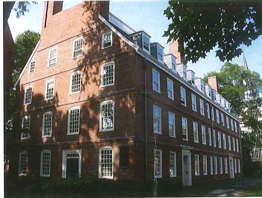
East and North Facades
