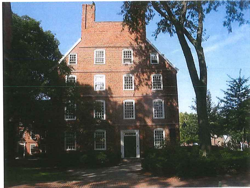
East (Yard) Facade
