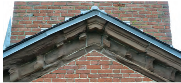
EXISTING EAST BROWNSTONE GABLE
