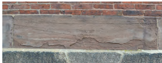
EXISTING SOUTH BROWNSTONE WATER TABLE
