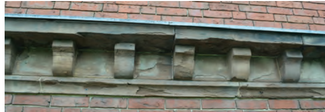
EXISTING SOUTH BROWNSTONE CORNICE
