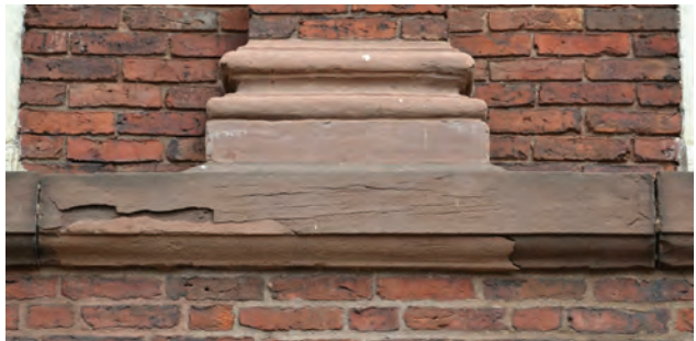
EXISTING SOUTH BROWNSTONE SILL AND PILASTER BASE
