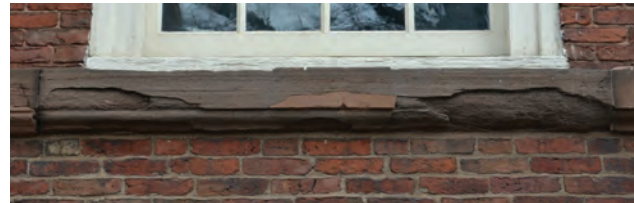
EXISTING SOUTH BROWNSTONE SILL
