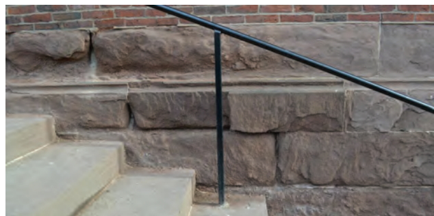
EXISTING SOUTH BROWNSTONE FOUNDATION
