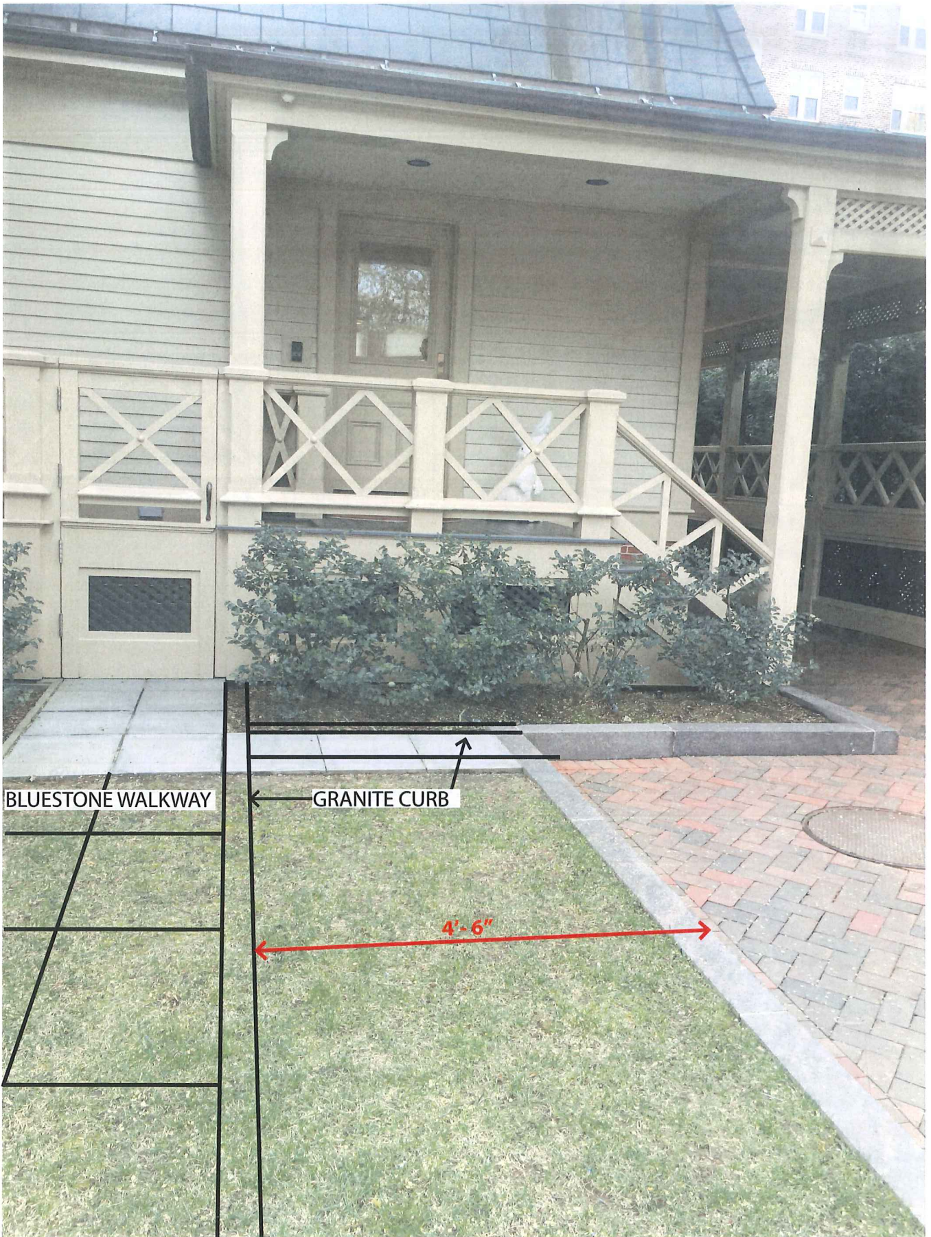
A: SHIFT CURB 4'-6" TO ALIGN WITH PORCH POST AND EXPAND BRICK DRIVEWAY
