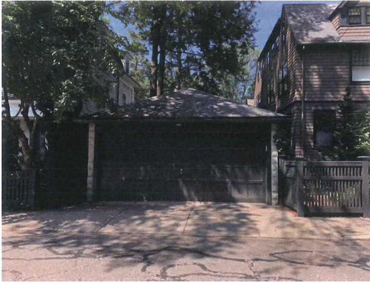
126 Brattle garage 8.15.19 existing conditions
