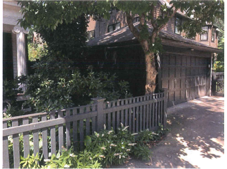
126 Brattle garage 8.15.19 existing conditions
