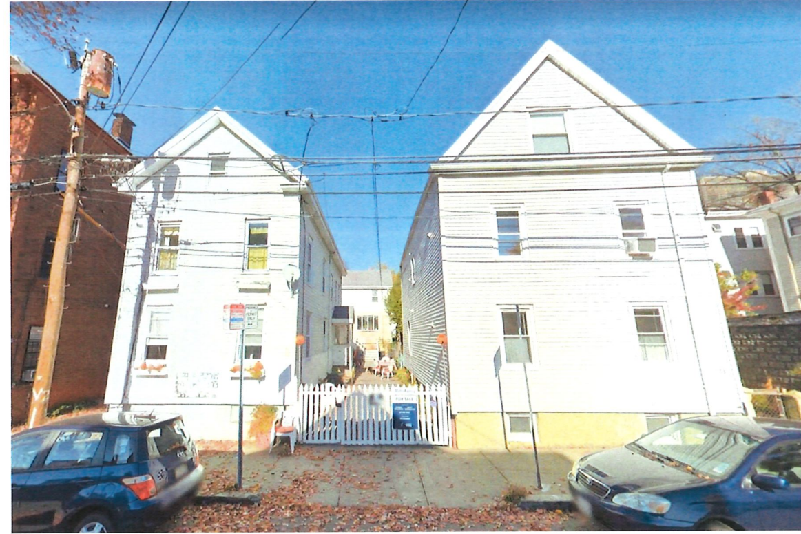
VIEW OF EXISTING SINGLE FAMILY FROM CHARLES STREET
