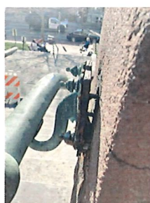
25 Upper Stair Railing - East A3.21
