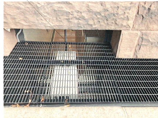
D West Facade - Window B Photo Scale:
