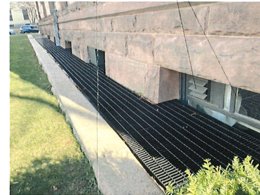
F West Facade - Window A'L Photo Scale:
