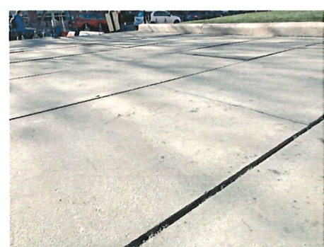
2 Landing Pavement Photo A3.20
