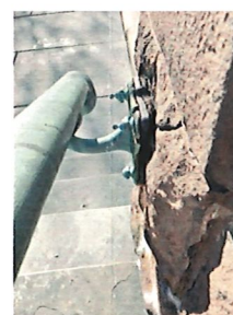
26 Upper Stair Railing Right A3.21
