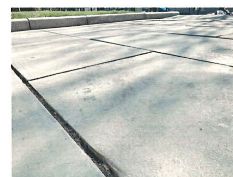
1 Landing Pavement Photo A3.20
