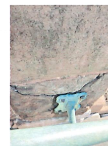
28 Lower Stair Railing - East A3.21
