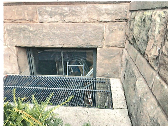
E South Facade - Basement Window at Infill Scale:
