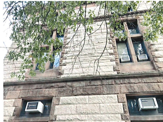
A West Facade - Window L Photo Scale:
