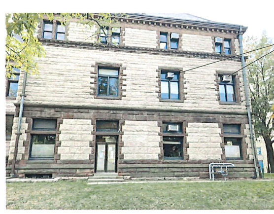
A North Facade - Photo Scale:
