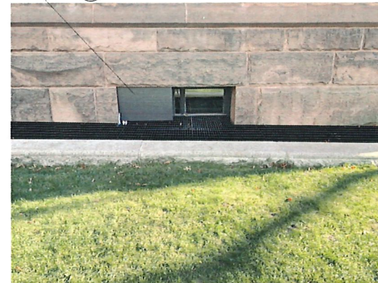
E West Facade - Window A' Photo Scale:
