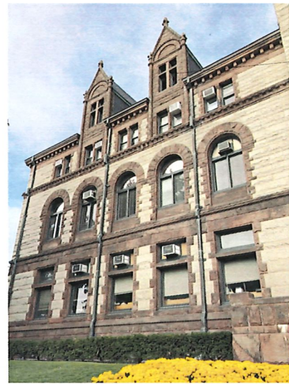
A South Facade - West Side Photo Scale:
