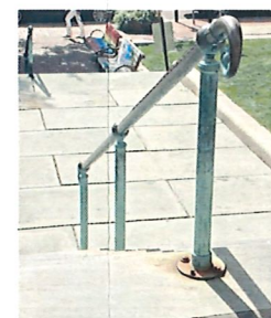
29 Upper Stair Railing - Middle A3.21
