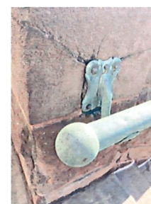
27 Upper Stair Railing - East A3.21
