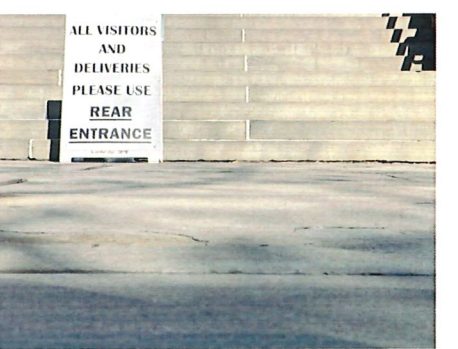
4 Landing Pavement Photo A3.20
