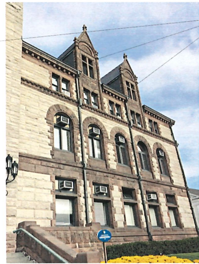
B South Facade - East Side Photo Scale:
