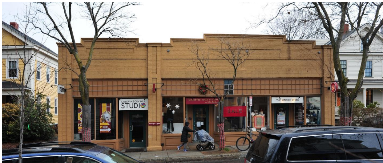
229 Concord Avenue (left), 221-225 Concord Avenue, and 219 Concord Avenue (right)
