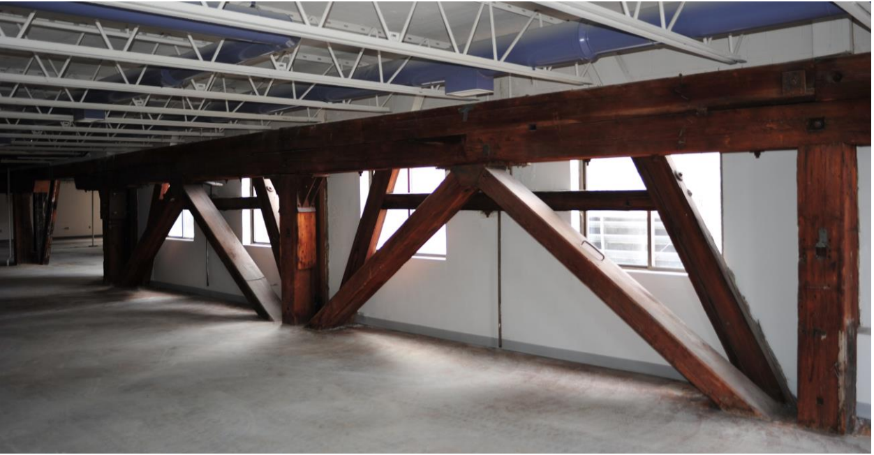
101 Rogers Street, third floor. Craneway framing.
