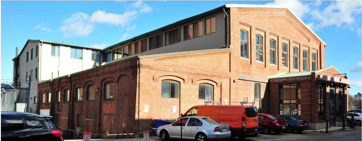
101 Rogers Street, west and south elevation
