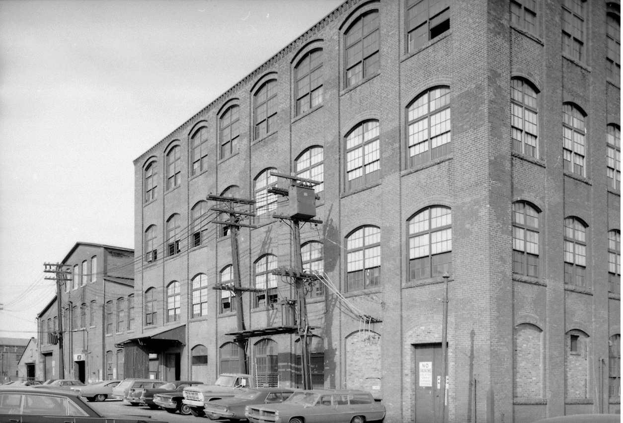
101 Rogers Street, 1969. The former pattern shop at right was razed in 1970.
