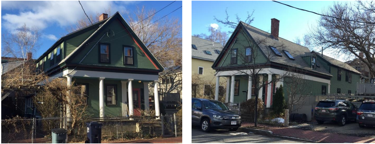
40 Cottage Street. North/front elevation (left) and west elevation (right). CHC photos 2017, 2018.
