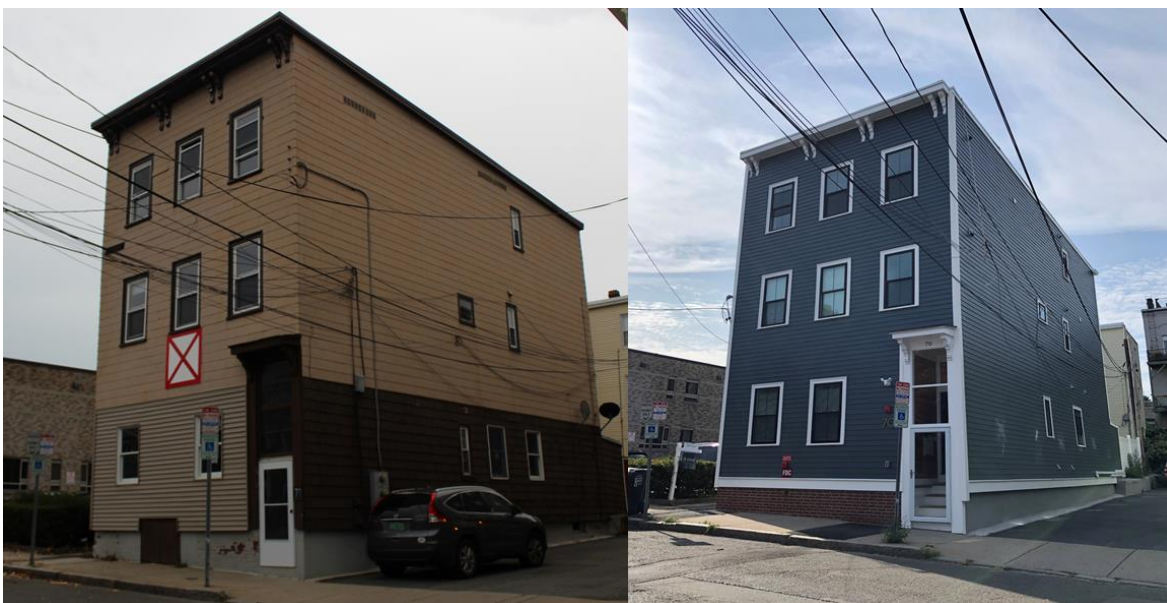
Case 4211: 70 Gore Street (1870) before and after administrative permit review.
