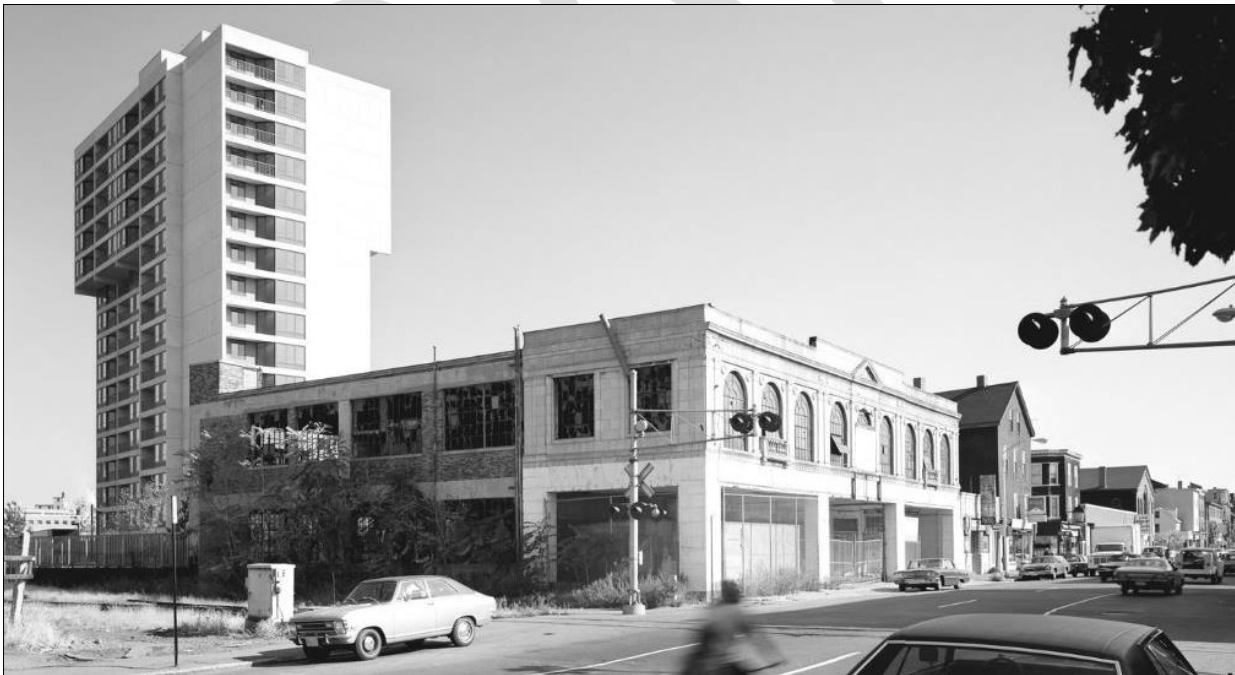
Cambridge Street looking east from the railroad crossing, 1974
