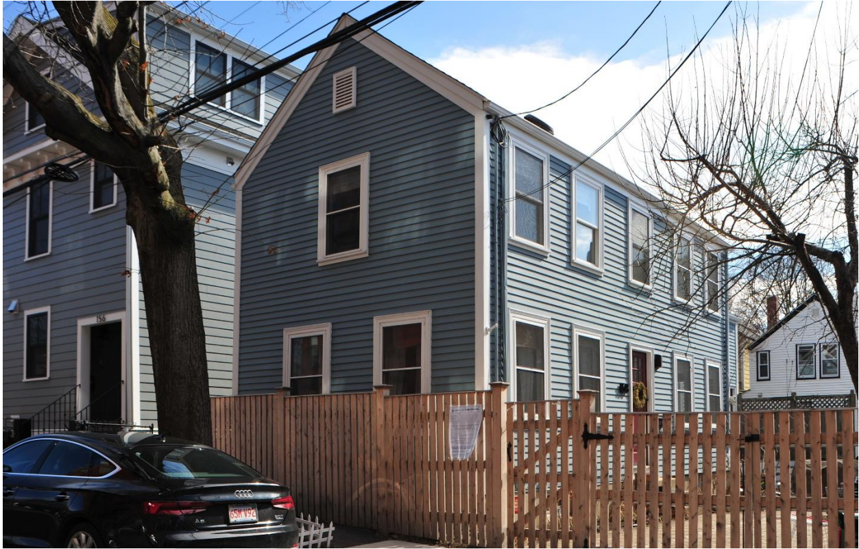
158 Thorndike Street before renovation.
