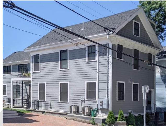
156 Thorndike Street as completed, showing removal of cornice brackets and random placement and sizes of windows. CHC staff photo, July 2022
