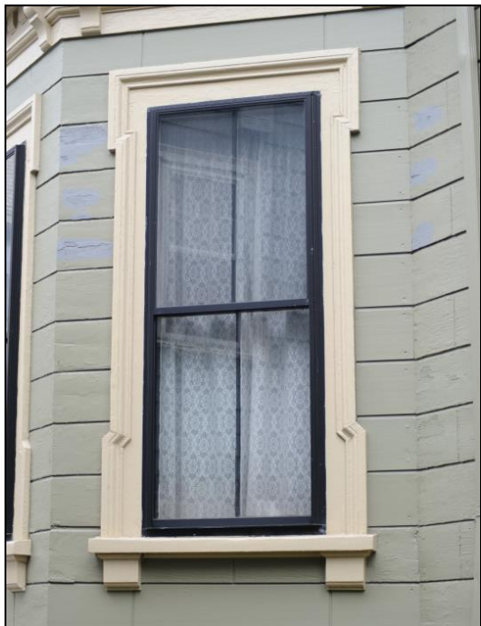
Figure 5: A restored double-hung wood window with a new storm window helps maintain the historic character of a building
