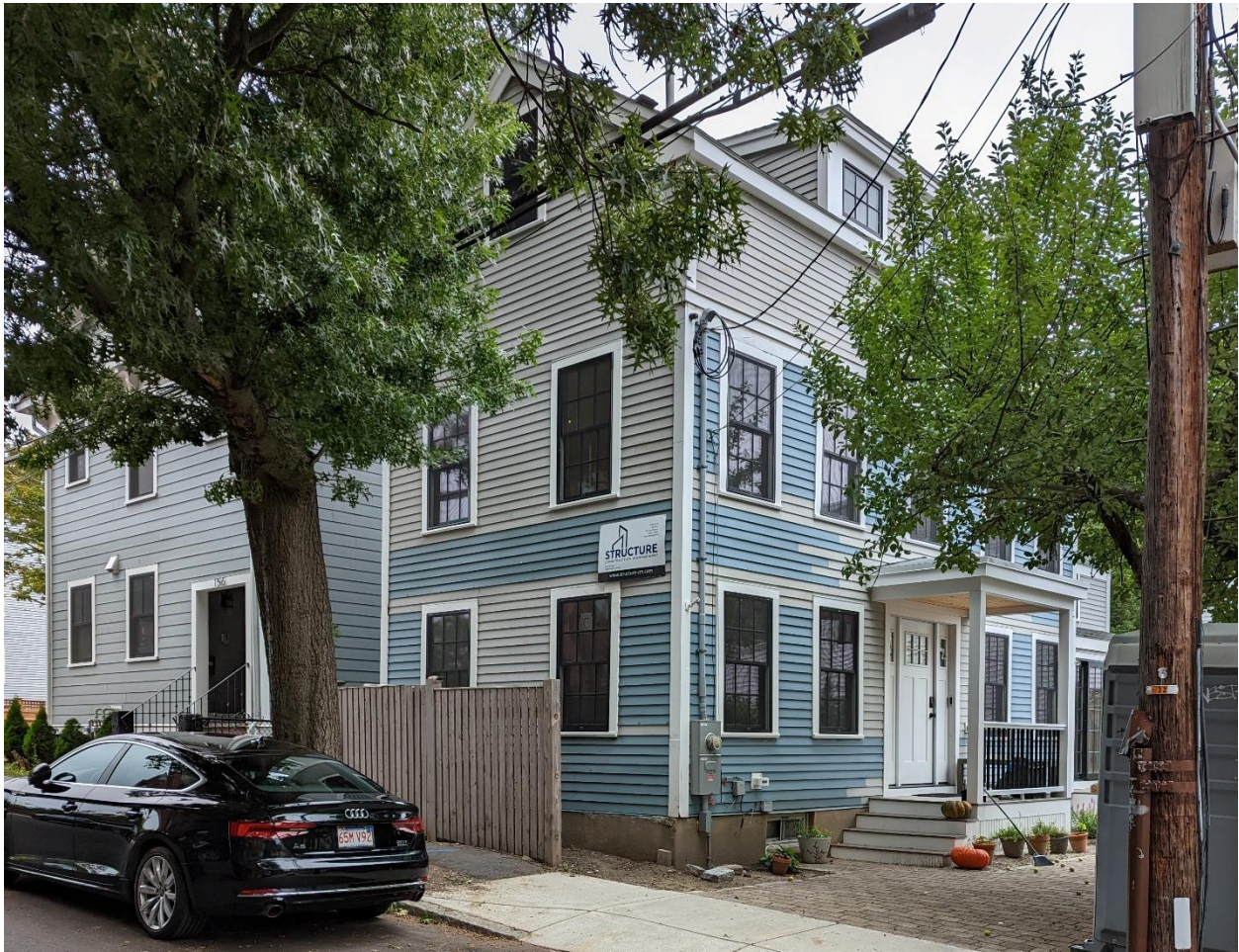
158 Thorndike Street, with renovation in process.
