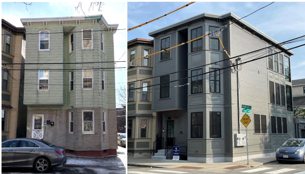
Case 4280, 66 Hurley Street (1907), before and after a renovation project that was granted a Certificate of Appropriateness in 2019. CHC photos, 2019 and 2021
