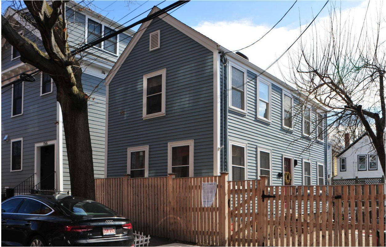
158 Thorndike Street before renovation.
