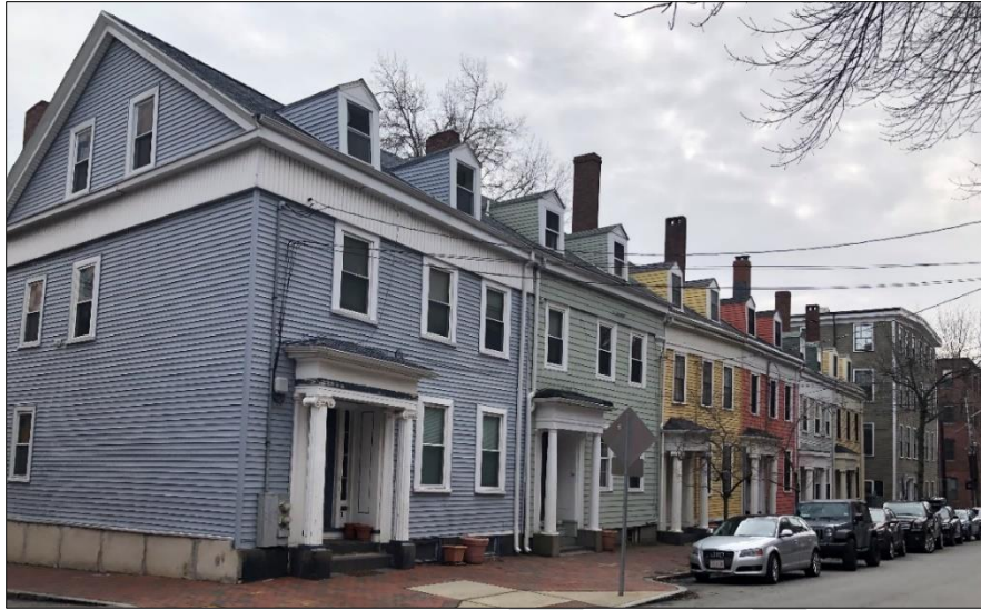
Greek Revival rowhouses (1842) at 36-46 Second Street
