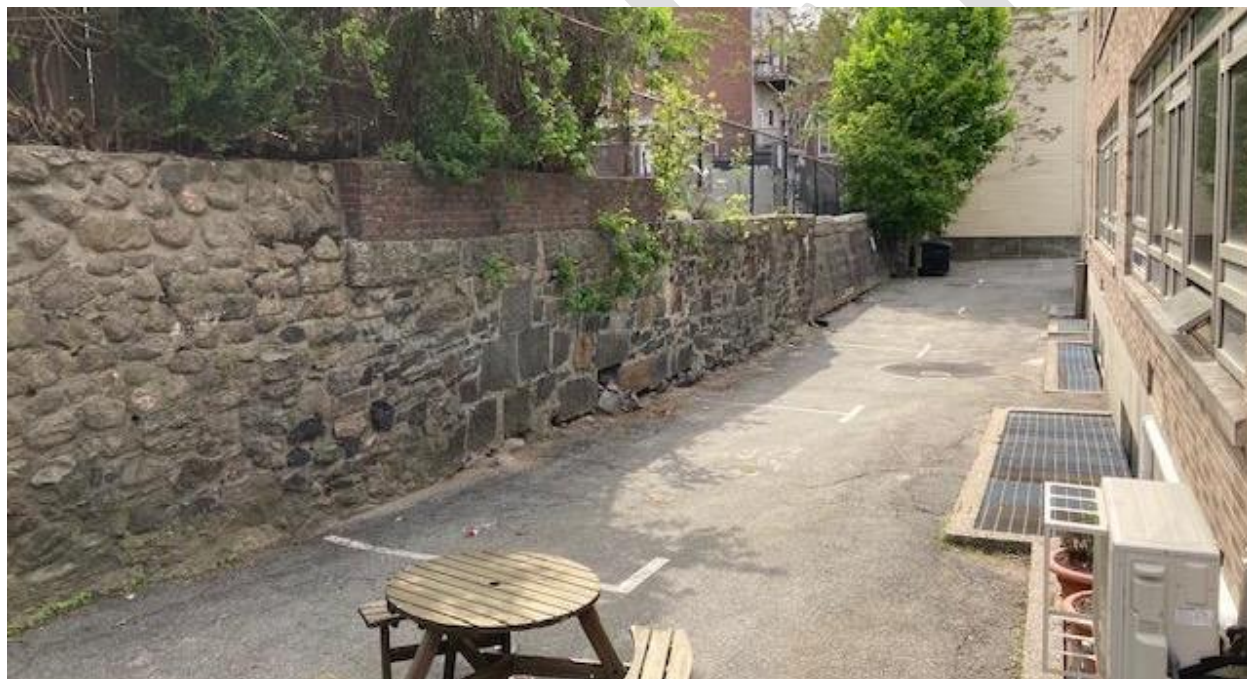
Stone and brick retaining wall at 60 Gore Street, possibly associated with the construction of the Gore Primary School in 1871. Destroyed 2022.
