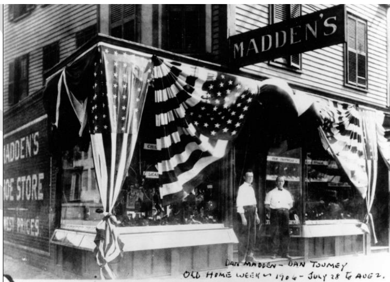
635 Cambridge Street (1867) with new storefront, 1906 CHC
