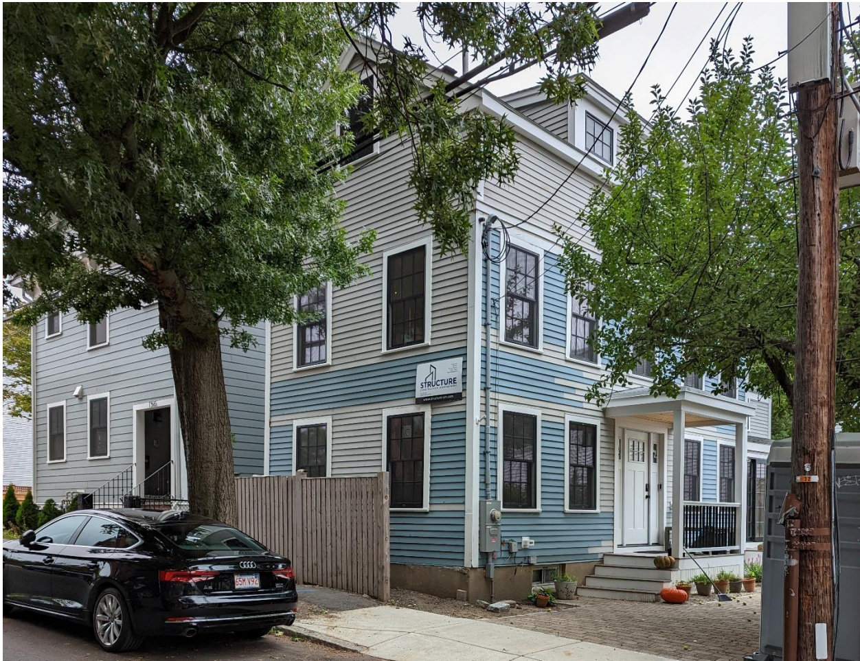
158 Thorndike Street, with renovation in process.
