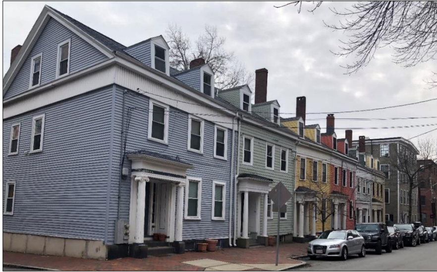
Greek Revival rowhouses (1842) at 36-46 Second Street
