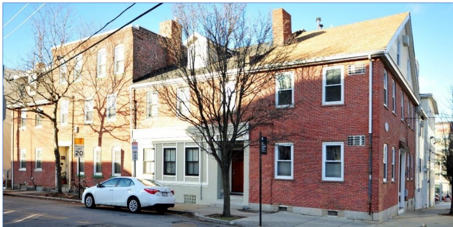
Lechmere Point Corp. houses (1821), 45-51 Gore Street. The two units on the right show the original roof form.
