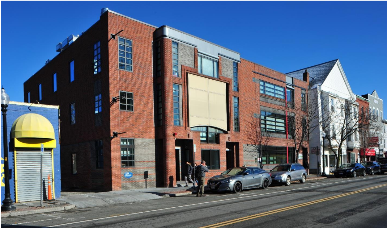
Former Hastings-Tapley Building, 271 Cambridge Street (1984), after renovation
