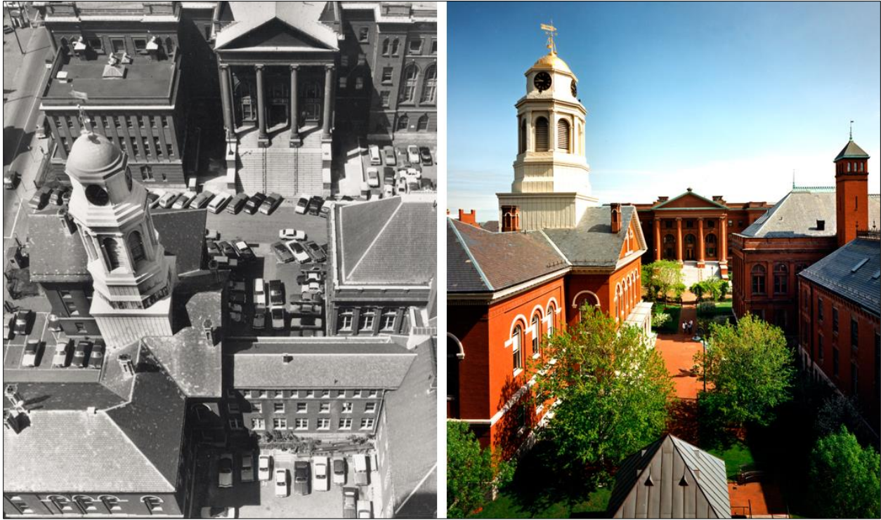
Middlesex County Complex – Bulfinch Square before and after 1984 restoration by Graham Gund.
