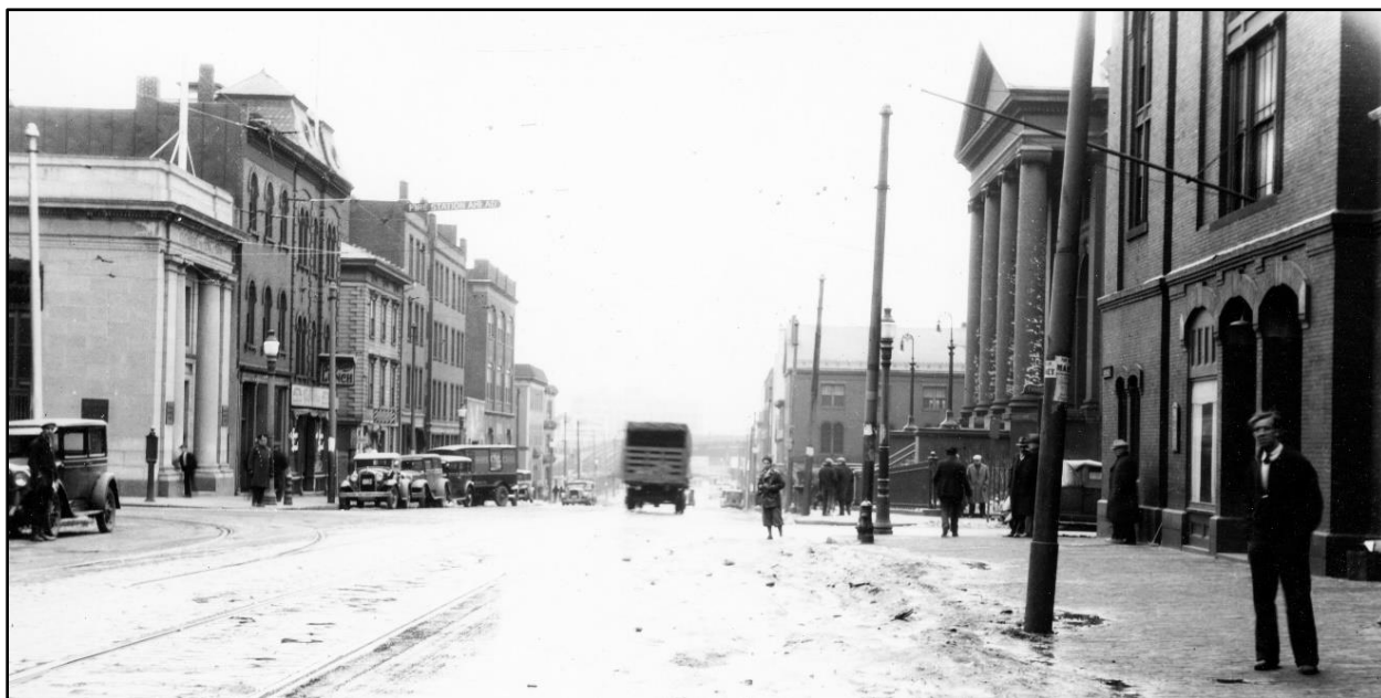
Cambridge Street at Third Street, looking east in 1934
