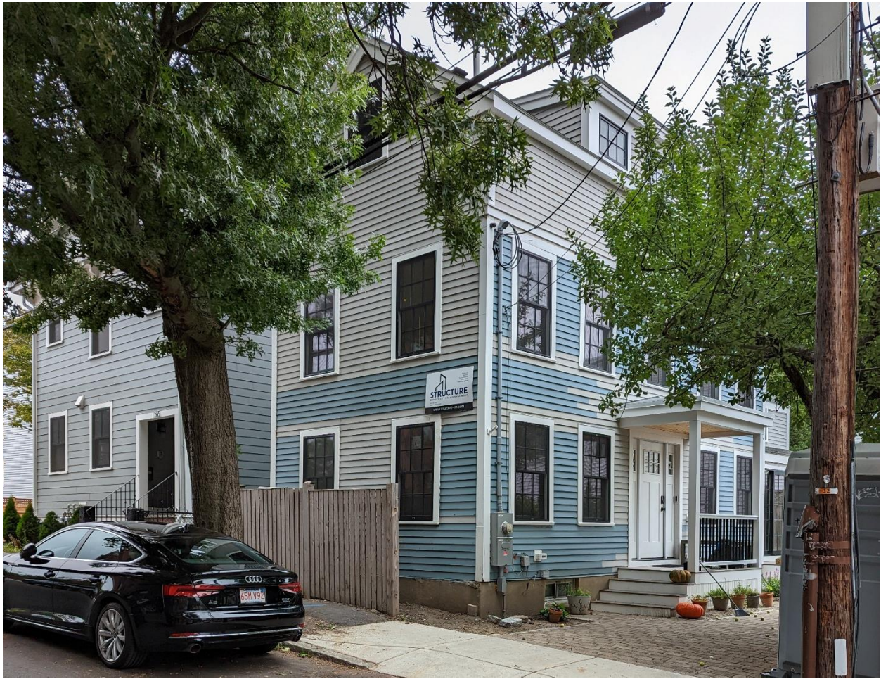
158 Thorndike Street, with renovation in process.
