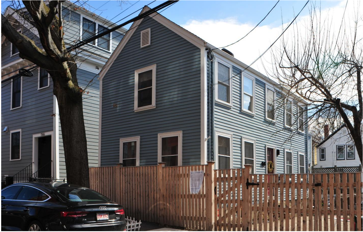
158 Thorndike Street before renovation.
