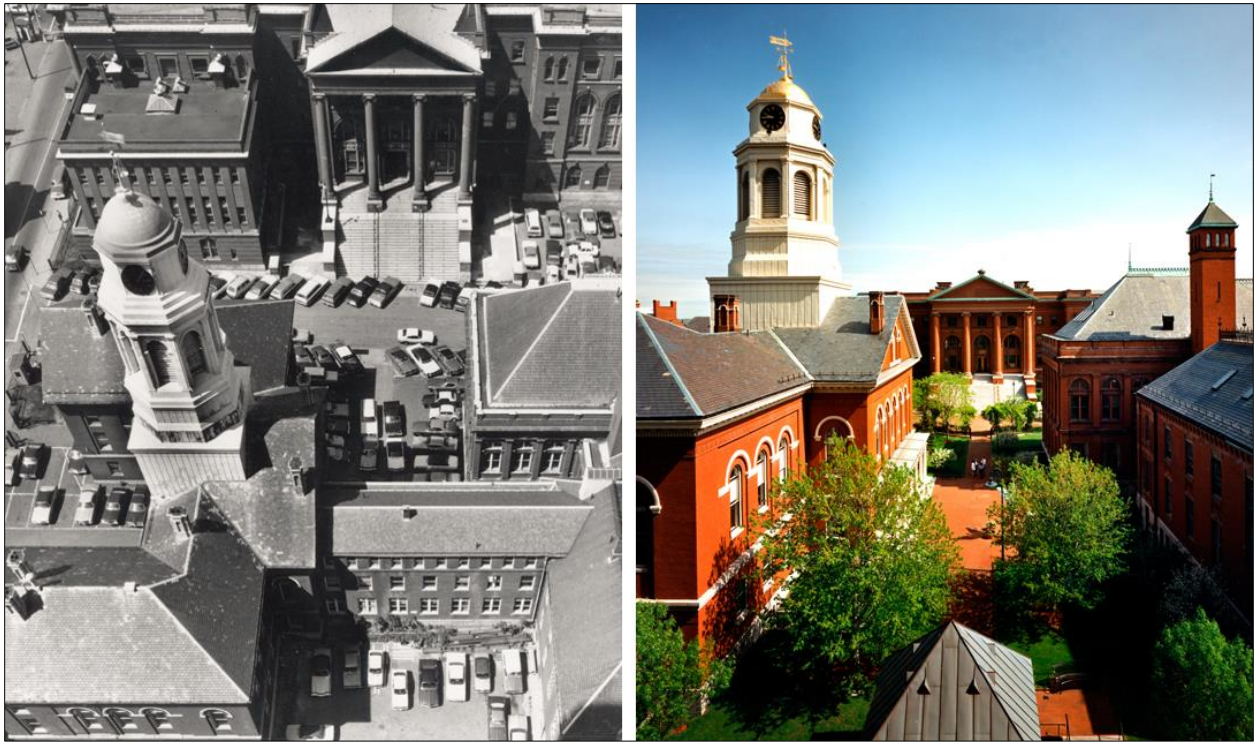
Middlesex County Complex – Bulfinch Square before and after 1984 restoration by Graham Gund.
