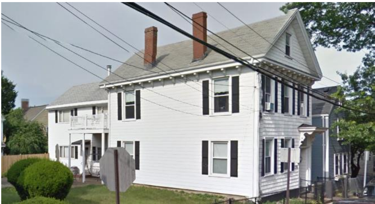
156 Thorndike Street with side porch removed, 2014
