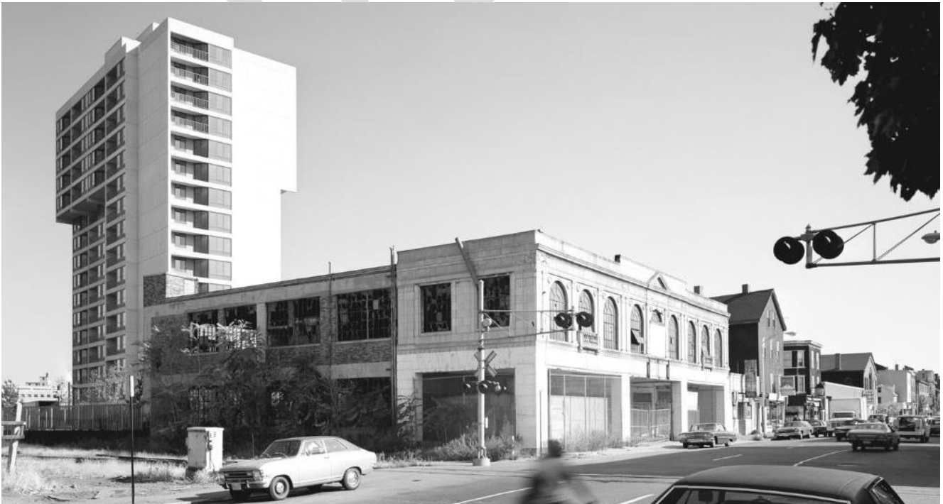
Cambridge Street looking east from the railroad crossing, 1974
