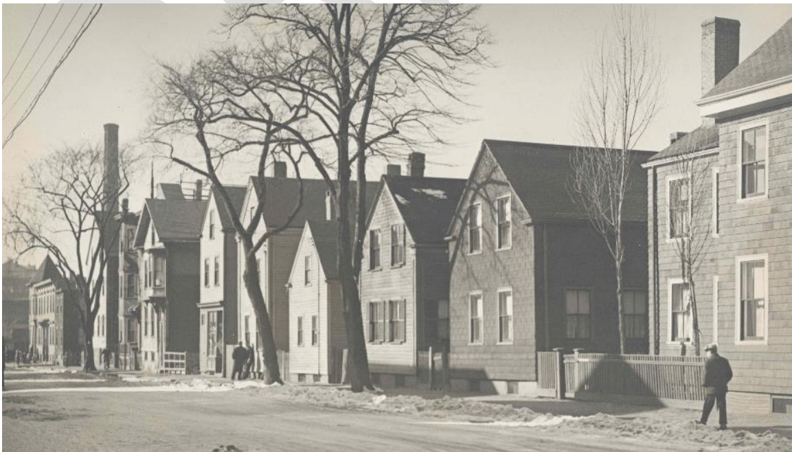
Winter Street Worker's Cottages, c.1940
