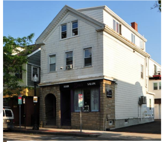
450 Cambridge Street (1856) with inserted storefront from 1901.
