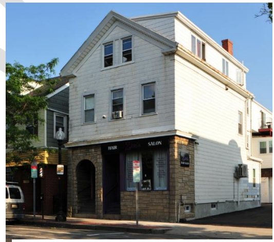
450 Cambridge Street (1856) with inserted storefront from 1901.
