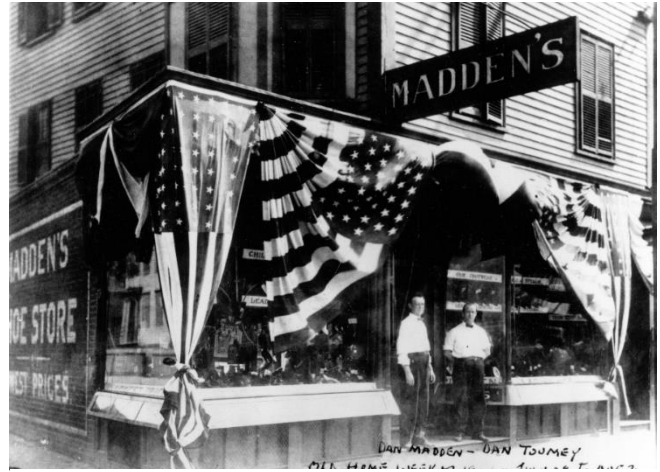
635 Cambridge Street (1867) with new storefront, 1906.
