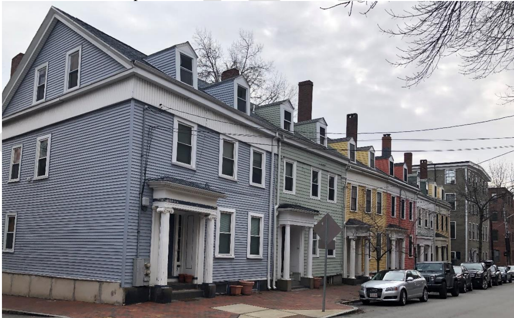
Greek Revival rowhouses (1842) at 36-46 Second Street
