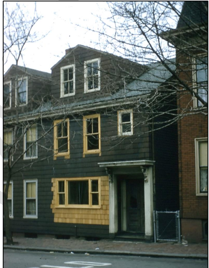
137 Otis Street ca.1946, with recently added picture window.
