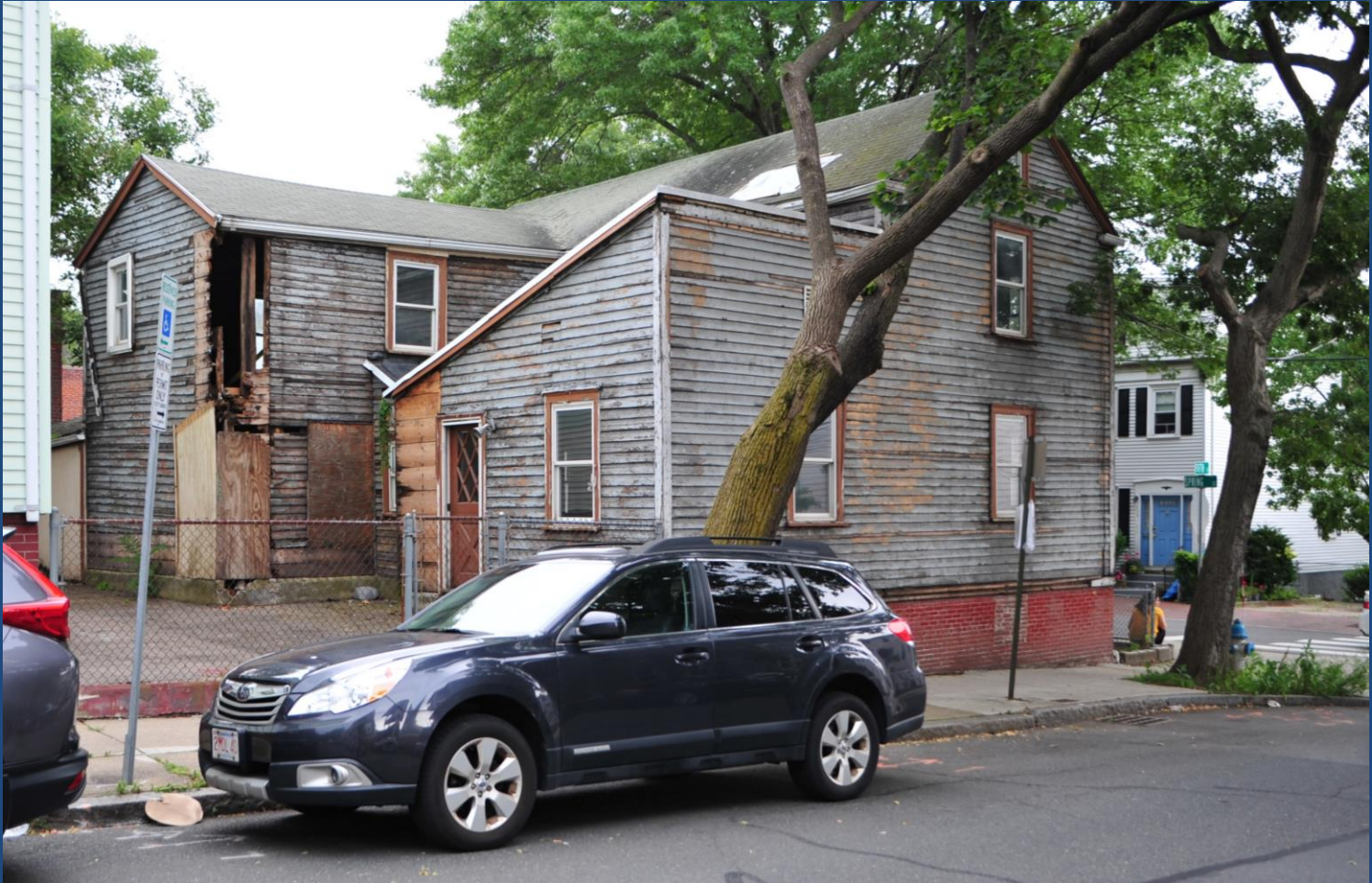
115 Spring Street (1826). Ells found not significant, 2019
