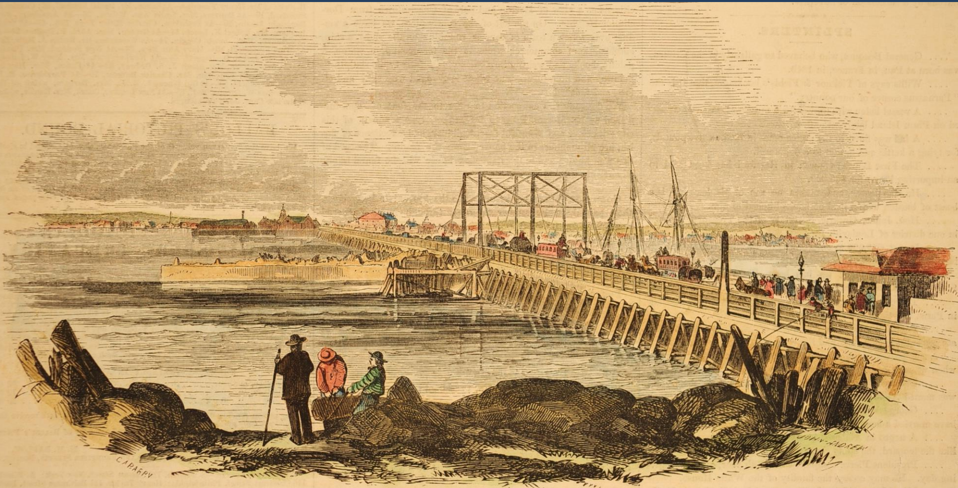
THE NEW CAMBRIDGE BRIDGE, BOSTON, MASS.
