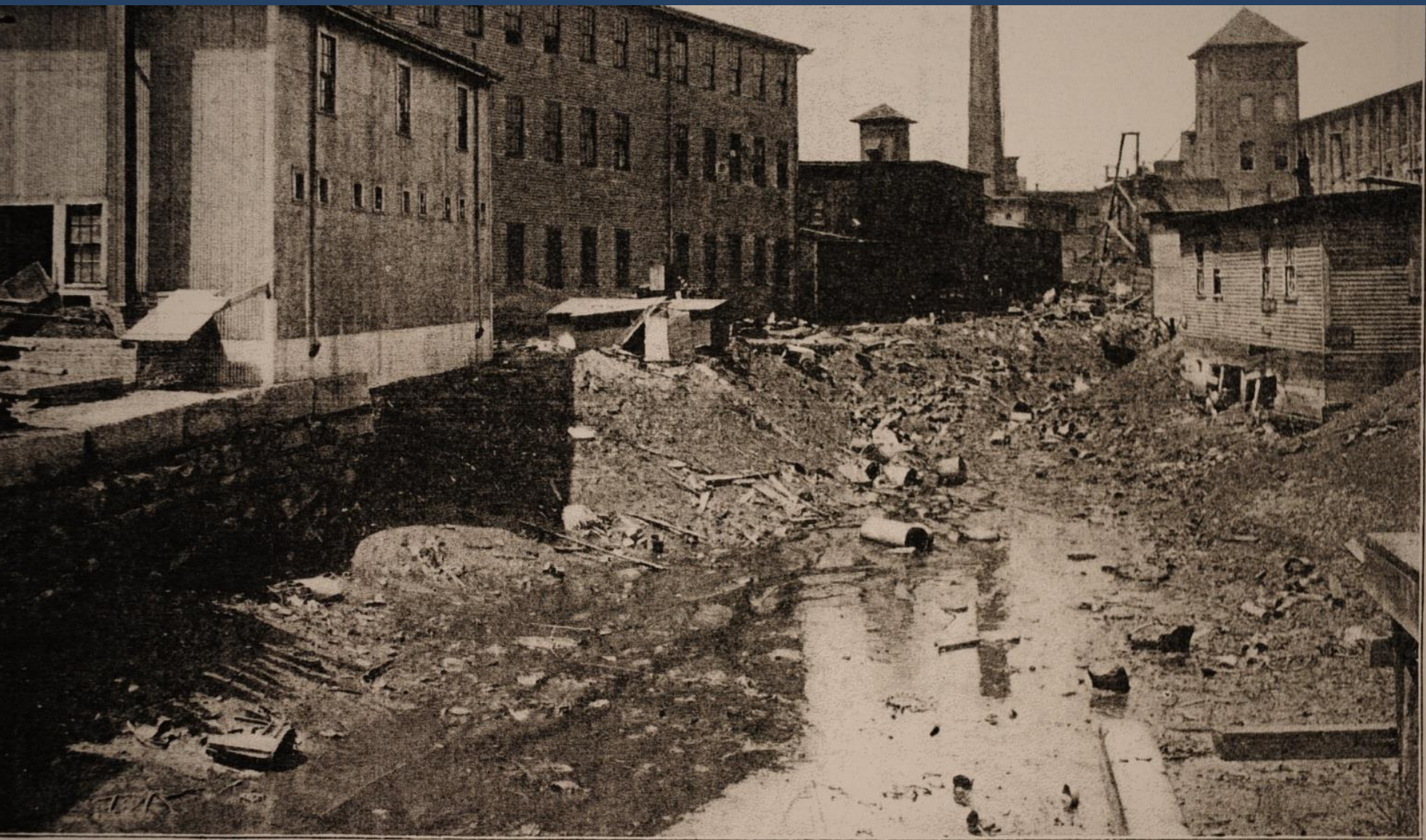
BROAD CANAL ABOVE RAILROAD BRIDGE, LOW WATER.
