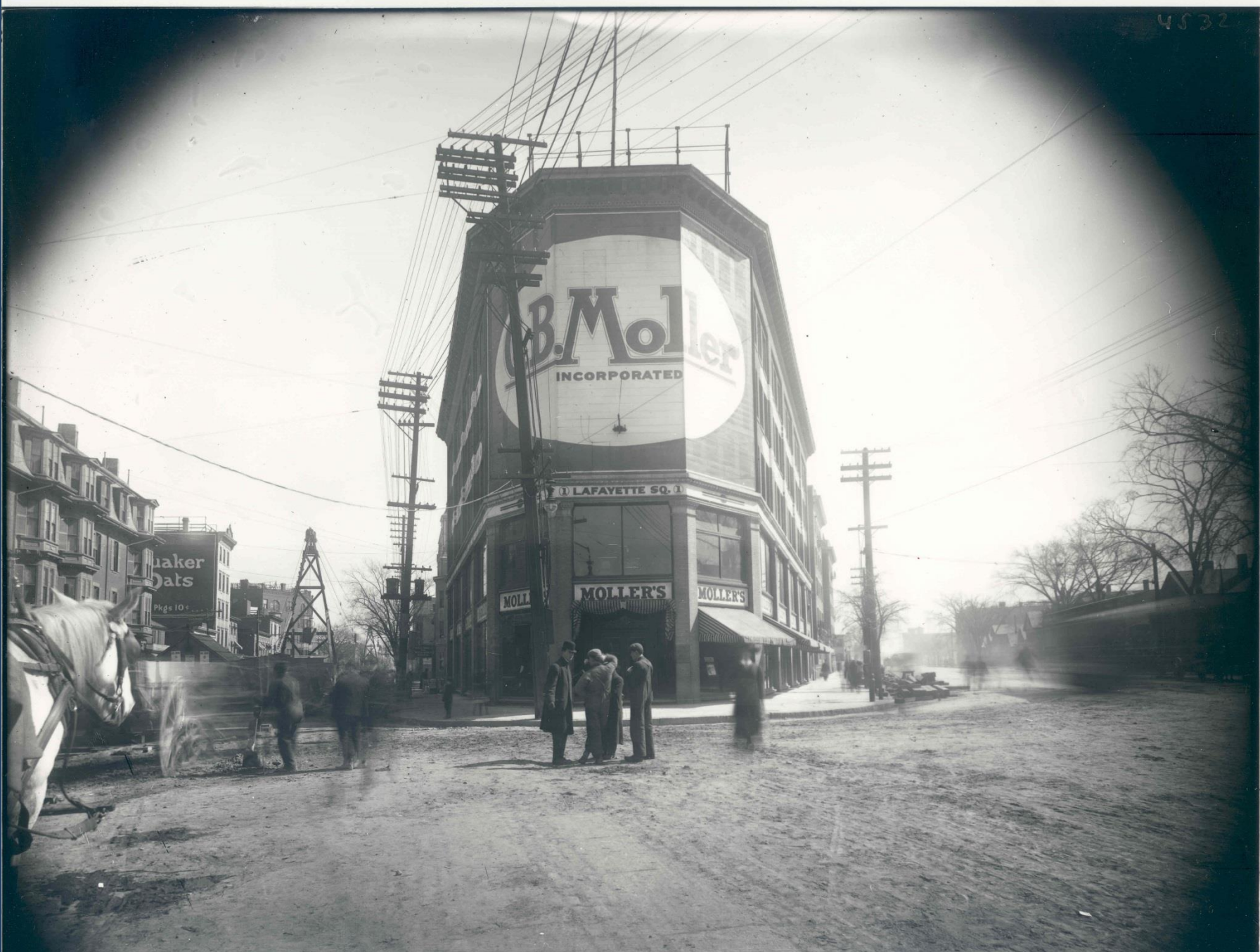
Moller Building, Junct. Mass. Av. and Main St
