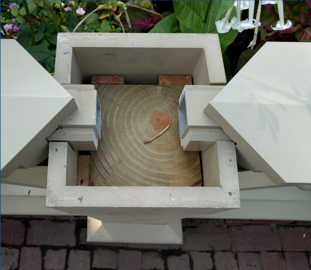
8 Follen Street, details of post and top rail PVC construction Contractor: Perfection Fence, Marshfield, Mass.
