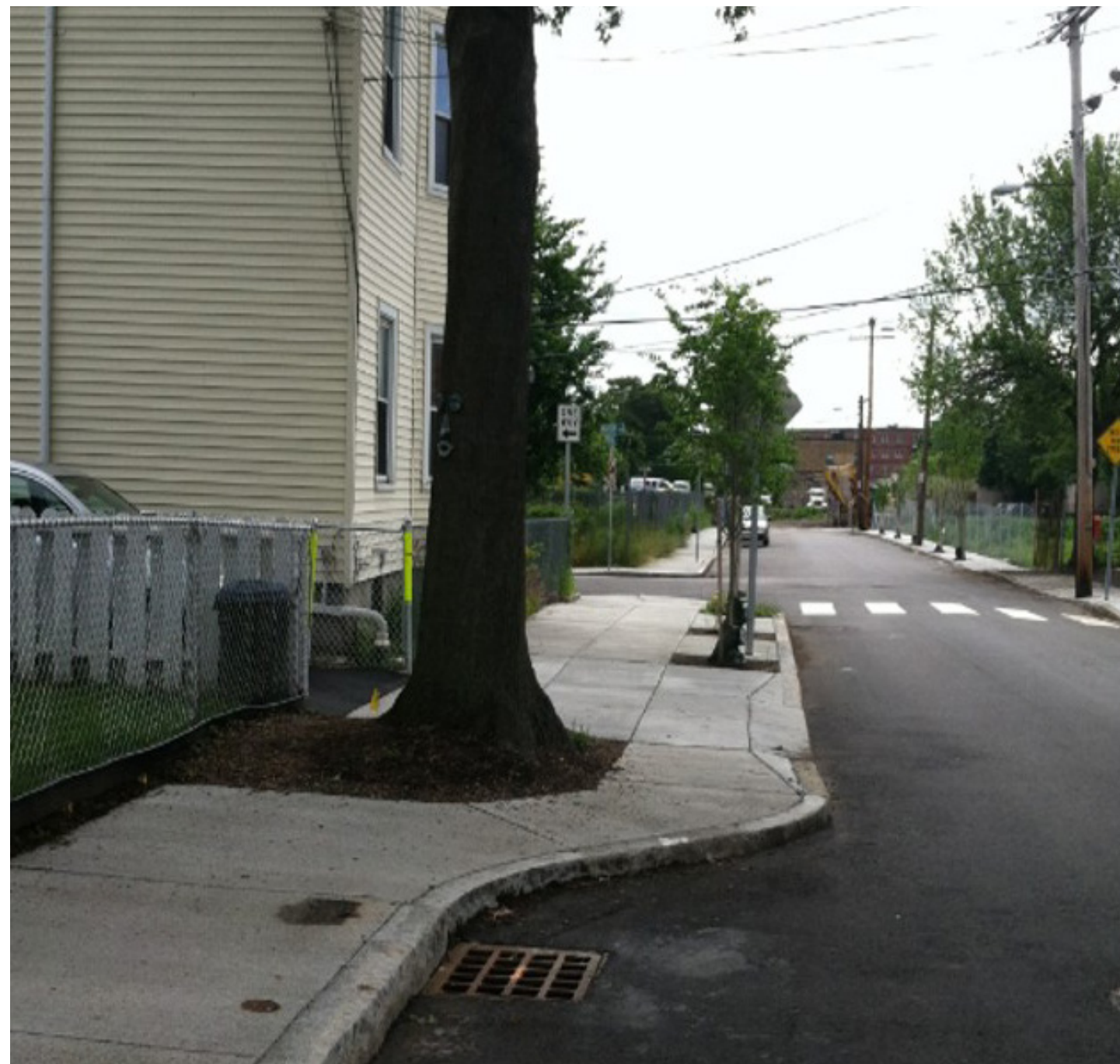
Curb Extensions for Accessibility
