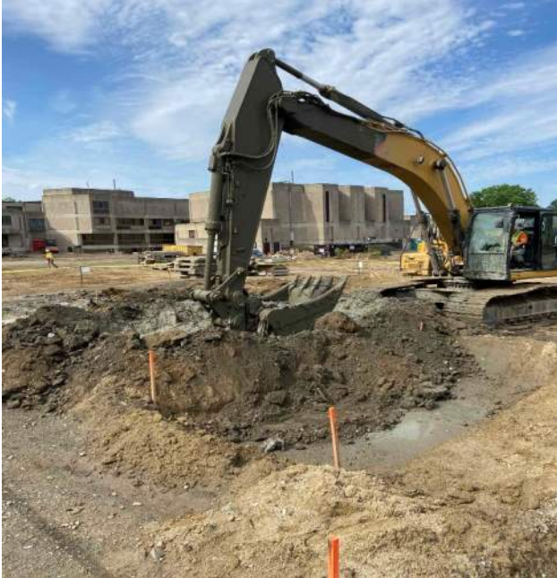
Ongoing Construction Soilcrete Wall, Insitu Soil Stabilization - Pilot Test
