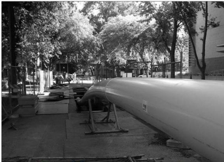
Insertion of slipliner from AWWA M28.
