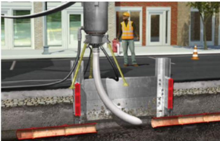
CIPP installation using inversion. Photo courtesy of InsituForm.
