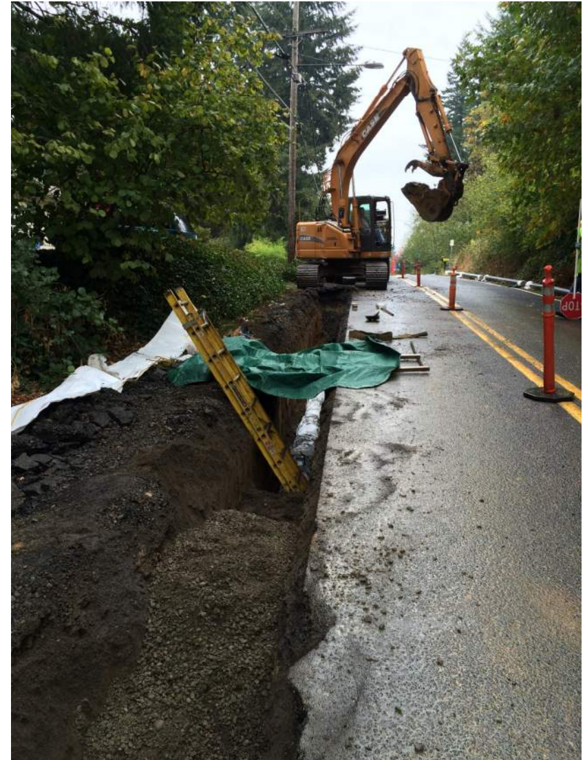
Example of open trench construction. Photo obtained at https://wedigportland.com/work-in-progress-flavel-watermain-improvement/
