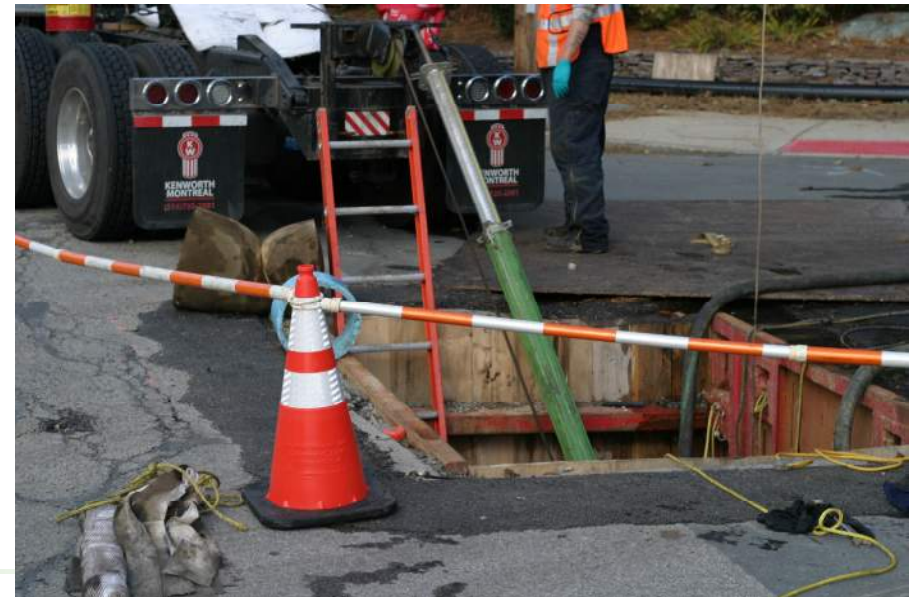
Example of trenchless rehabilitation with HDPE. Photo obtained at https://wedigportland.com/work-in-progress-flavel-watermain-improvement/
