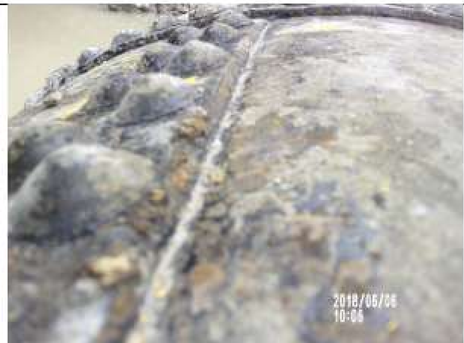
Pipe close-up of rivet seam
