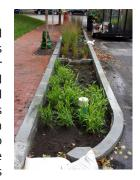
are washed off the land surface with the first 1/2" to 1" of runoff. The goal for biobasins is to intercept and treat the first inch of pavement runoff, known as the "first flush".
