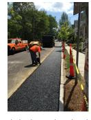
to the City's storm drain system and discharged to local waterways. Similar to biobasins, the City's goal for porous pavement is to intercept and treat the "first flush" of runoff.
