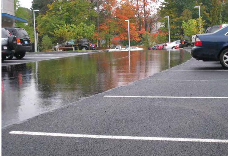
**Figure 7: Porous Asphalt Parking Stalls**
