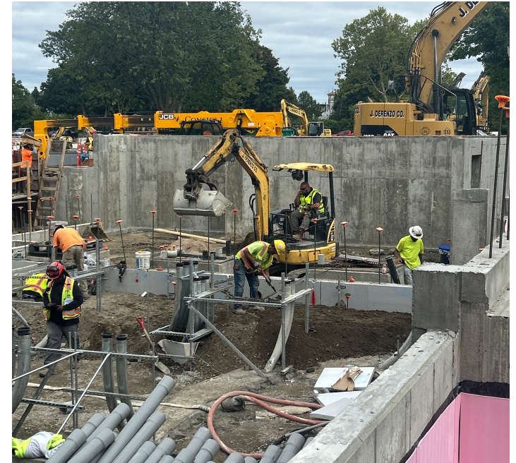
Active construction of Jefferson Park Federal
