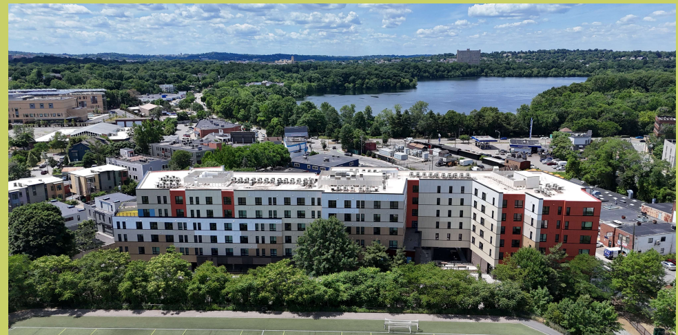
Pictured: Aerial view of 52 New Street completed
