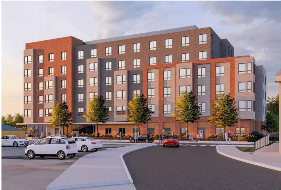
87-101 Blanchard Road (now under construction)
