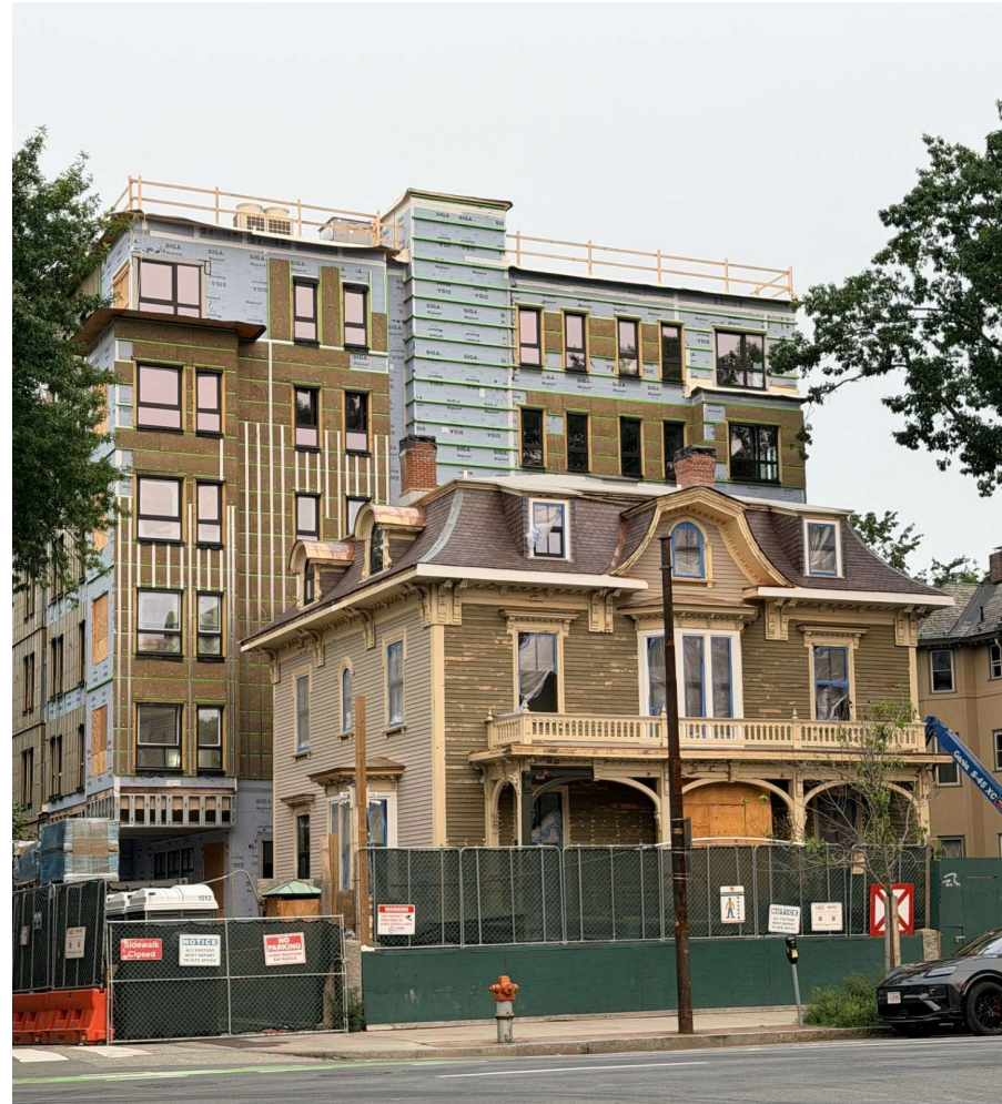
4 Mellen Street (under construction)
