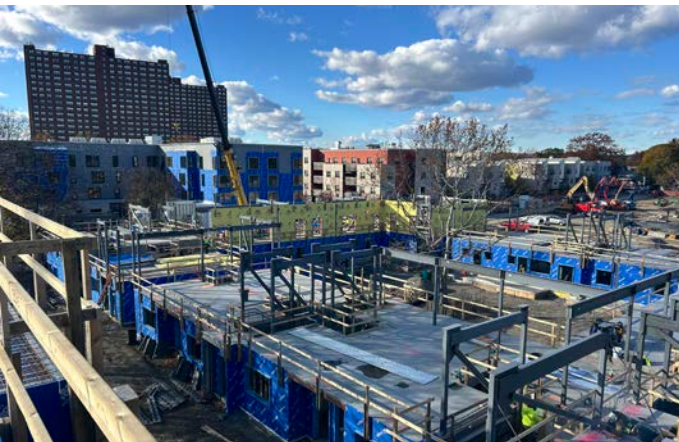
Jefferson Park Federal, North Cambridge, 278 units — Status: under construction.
