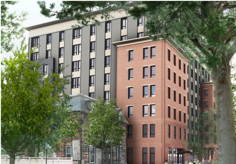
Rendering of 28-30 Wendell Street, Baldwin, 95 units — Status: preparing for construction.
