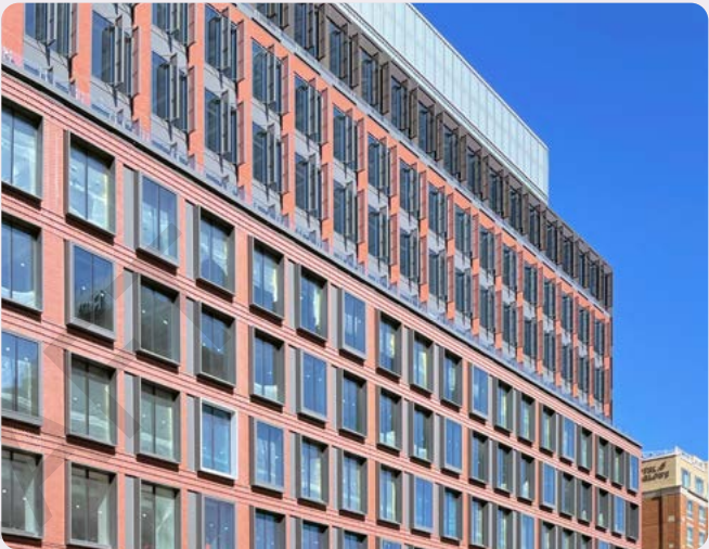
FIG. 67 20 Cambridgeside building facade features shading devices around glazed areas that will help enhance building performance by reducing cooling needs for tenants.
