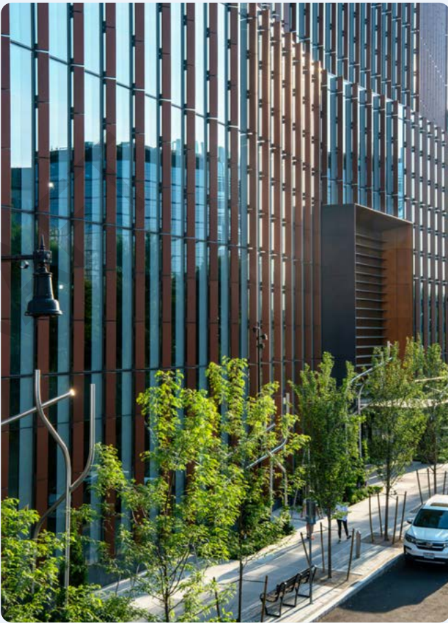
FIG. 27 This life science building on Morgan St. uses vertical fins to help mitigate glare.
