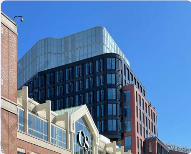
FIG. 62 The mechanical penthouse of the 20 Cambridgeside place development steps back from the floors below.
