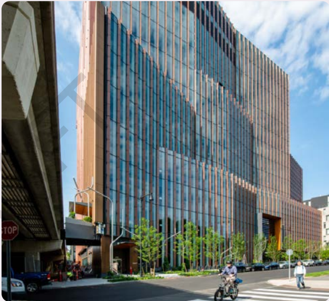
FIG. 76 The vertical fins on 411 Morgan Ave minimize glare and solar gain, while its orientation optimizes daylighting.
