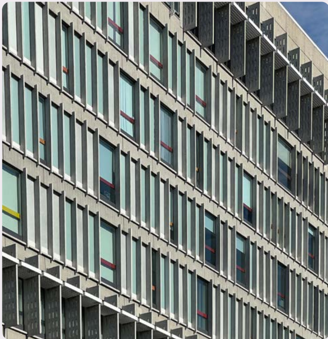
FIG. 79 Light-colored materials and sun shading devices above windows are passive design strategies that can help mitigate heat and maintain occupant comfort during power outages and extreme events.
