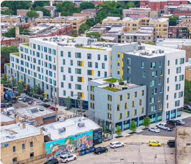
FIG. 87 The massing of this mid-rise residential building in Chicago steps down to relate to the height of nearby smaller-scale buildings.
