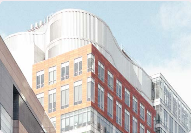
FIG. 83 Building on Ames St uses a curved wall to screen mechanical equipment, while adding visual interest to the building top.
