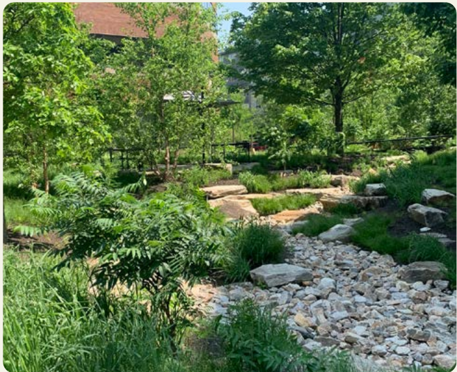
FIG. 117 Rain gardens manage stormwater in Alewife open space.
