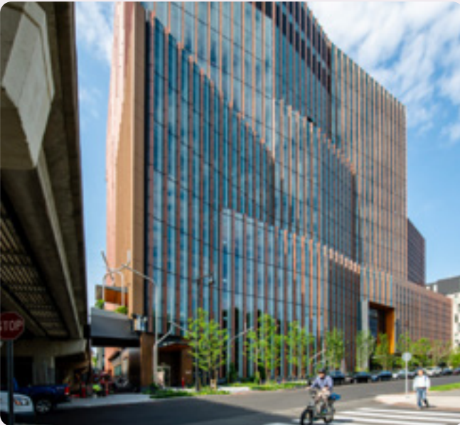
FIG. 81 The vertical fins on 411 Morgan Ave minimize glare and solar gain, while its orientation optimizes daylighting.
