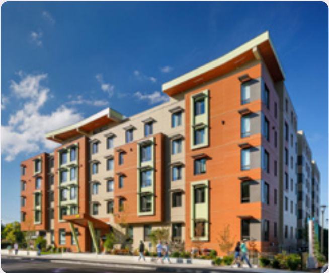
FIG. 83 Finch Cambridge uses heat exchange systems, highly insulative materials, and an airtight envelope, and earned a Passive House certification.
