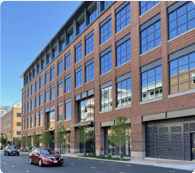
FIG. 60 The structural bays are expressed on the streetwall facade of the 60 First St building.
