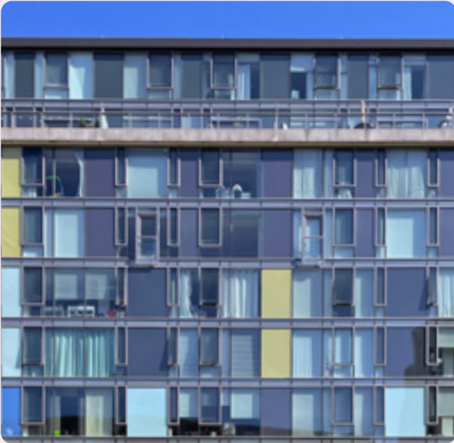
FIG. 77 A combination of transparent glazing, infill panels, and shadow boxes can balance visual connection with building energy performance. This material choice has both texture and pattern.
