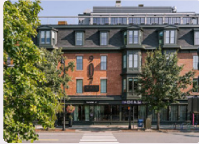
FIG. 79 The restoration of 907 Main St preserves original details and materials.
