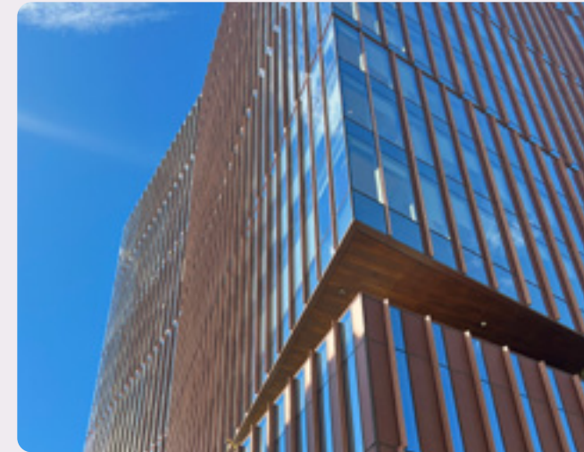
FIG. 63 Long, vertical fins on taller buildings emphasize height and help break up the horizontality of wider buildings.
