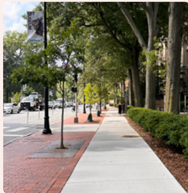
FIG. 202 Massachusetts Avenue sidewalks feature a defined Pedestrian Zone with poured concrete, complemented by a red brick edge in the Planting/Furnishing Zone.
