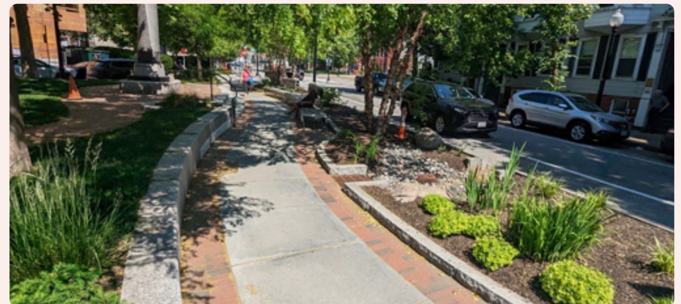
FIG. 201 Western Ave features a continuous planting bed with a raised curb, and green infrastructure and low plantings that protect street trees and vulnerable street users.
