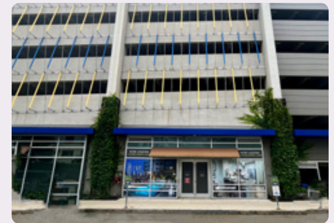
FIG. 98 Active ground floor uses are included in a parking garage.
