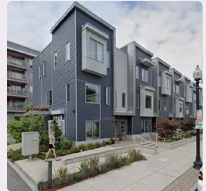
FIG. 54 Coppersmith Village in East Boston balances privacy and accessibility with a continuous accessible passage to individual unit entrances.
