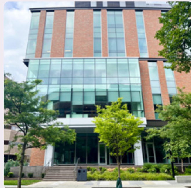
FIG. 56 This building's elevated first floor allows for the addition of plantings and an inviting streetscape.
