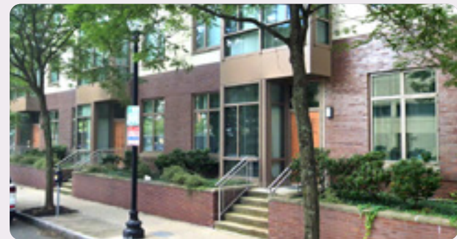
FIG. 53 The ground floor along Munroe St features frequent individual residential unit entrances.
