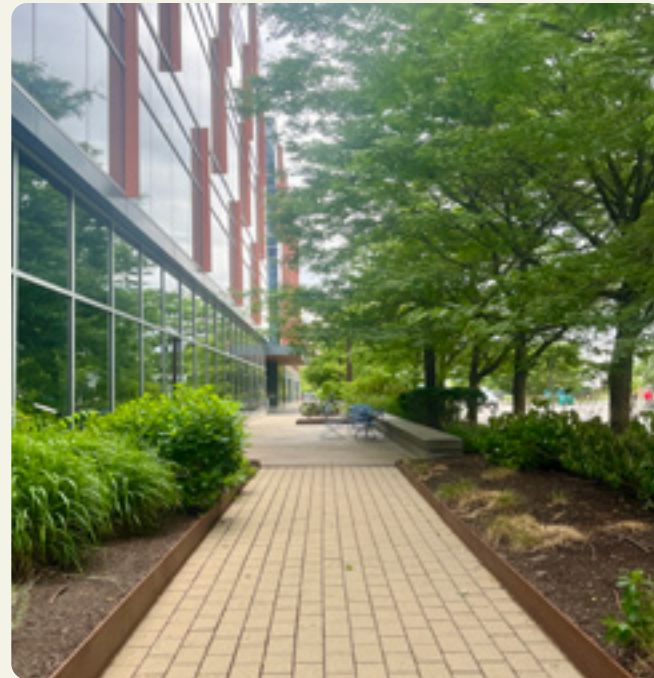
FIG. 132 A sidewalk in Alewife utilizes high SRI and permeable paving materials.
