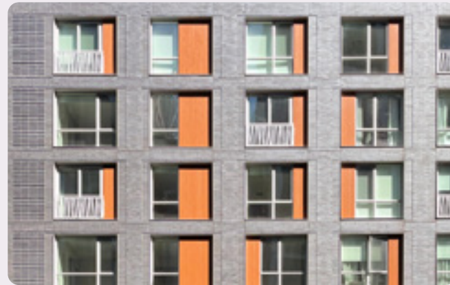
FIG. 71 Brick details, recessed windows with wood infill panels, and railings add rich detail and visual depth, creating an engaging façade.
