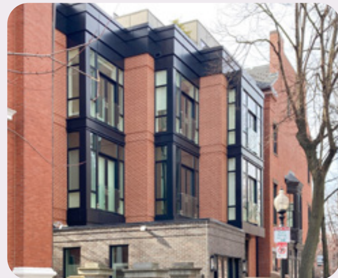
FIG. 74 Bay windows of this residential building feature windows on the sides in addition to the front face.
