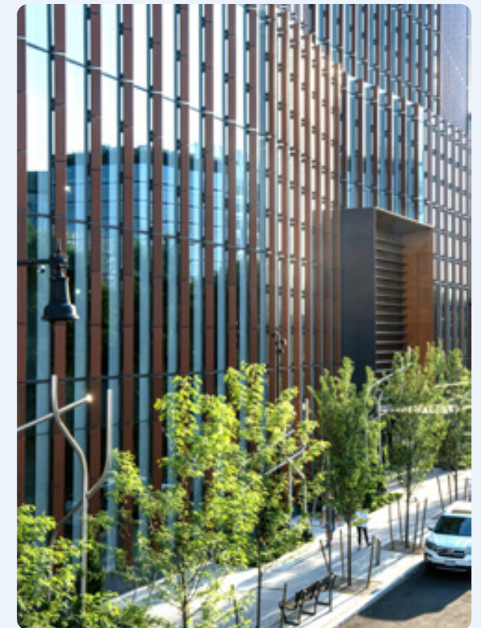
FIG. 29 Vertical fins at 441 Morgan Ave help diffuse glare, enhancing visual comfort and contributing to a more refined architectural expression.
