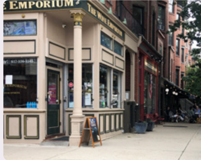
FIG. 46 Corner store in Boston's South End features windows on both street frontages.
