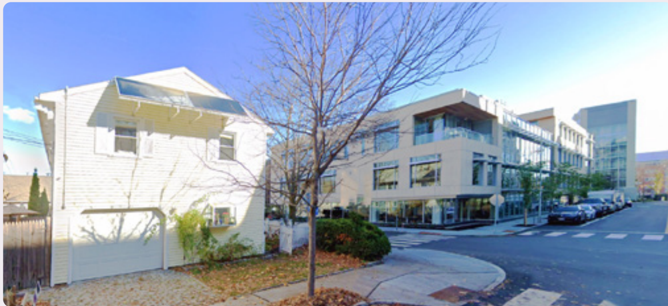
FIG. 36 A development near Kendall Square (right) uses massing, facade changes, and materials to create a sensitive transition to the nearby residential neighborhood (left).
