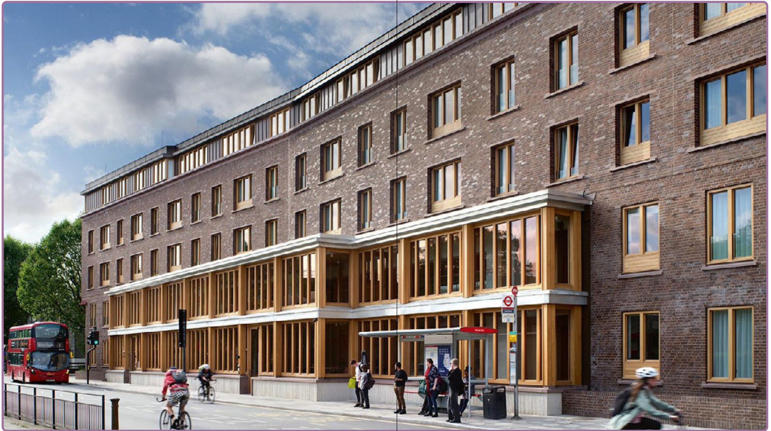
The Appleby Blue senior housing project in London, England features a four story brick principal facade with a stepped back top floor, and a two-story wood and glass projecting element on the lower floors. The organization of the massing in relation to the material changes enlivens the streetscape.
