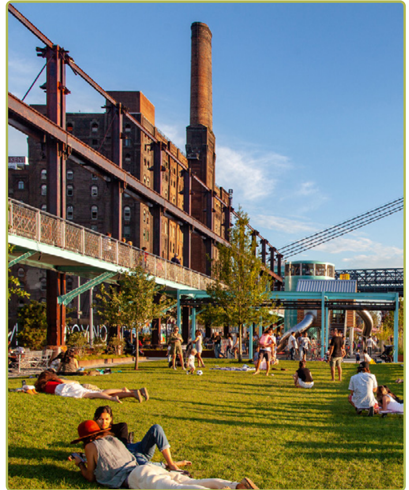
Domino Park in Brooklyn, NY incorporates the history of the former industrial waterfront into a riverfront park that serves the diverse community of New York residents and visitors. The park is raised above the floodplain and features native plant species that reduce stormwater runoff and provide protection from damaging storm surges.
