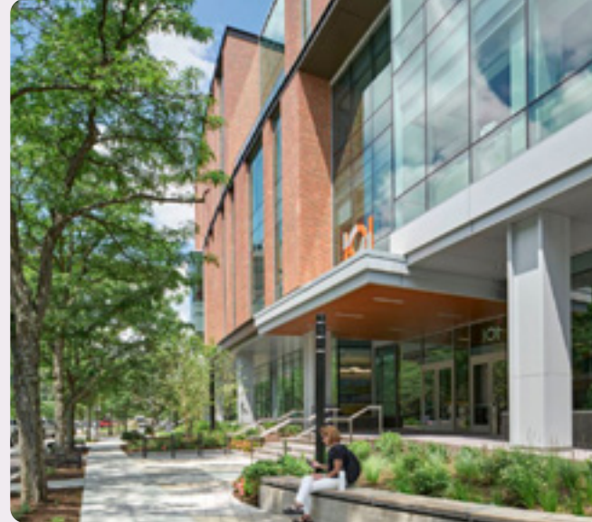
FIG. 50 A canopy provides shade in warm weather, protection from rain and snow, and visually celebrates the building's entry, enhancing both comfort and arrival experience.
