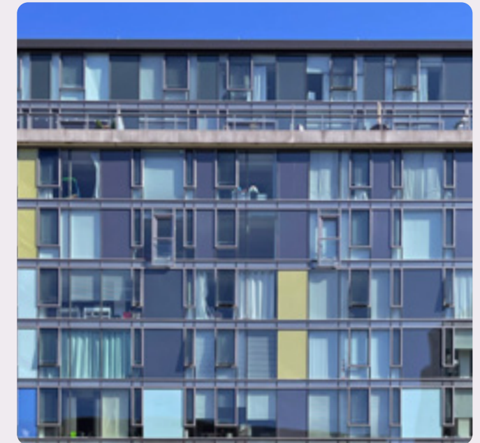
FIG. 77 A combination of transparent glazing, infill panels, and shadow boxes can balance visual connection with building energy performance. This material choice has both texture and pattern.
