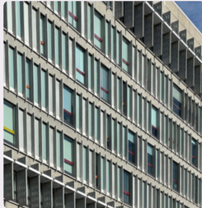
FIG. 84 Light-colored materials and sun shading devices are passive design strategies that can help mitigate heat and maintain occupant comfort during power outages and extreme events.
