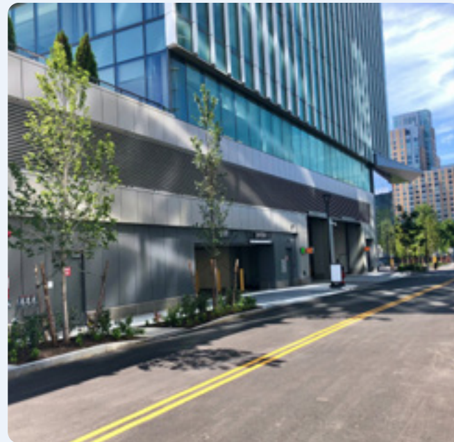
FIG. 22 Structured parking is accessed via an internal driveway at 450 Water St, strategically located away from the primary street to minimize disruption for people walking and biking.
