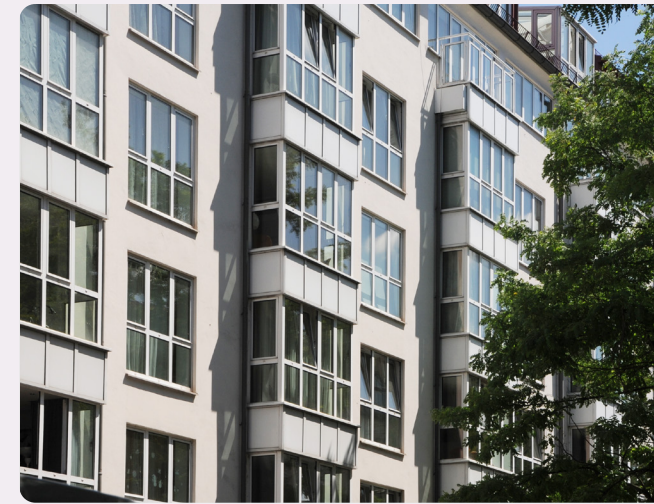
FIG. 95 Apartment building in Munich, Germany features multiple-pane bay windows in the facade.
