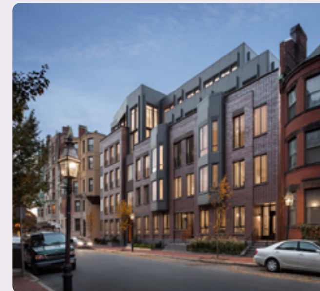
FIG. 93 The massing of this mid-rise residential building in Boston steps down to relate to the height of nearby smaller-scale buildings.
