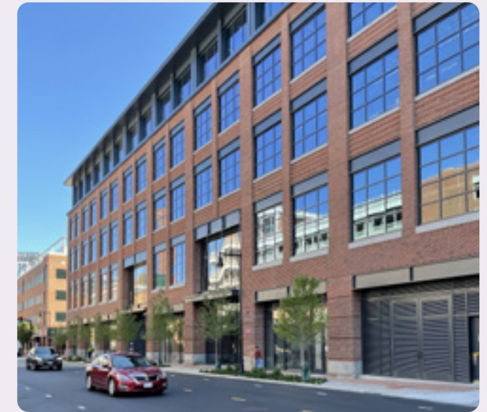
FIG. 60 The structural bays are expressed on the streetwall facade of the 60 First St building.
