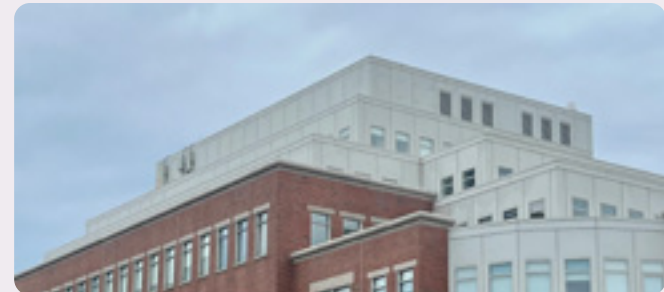
FIG. 90 Facade mounted antenna in Harvard Square avoid the principal brick facades and match the penthouse color and finish.
