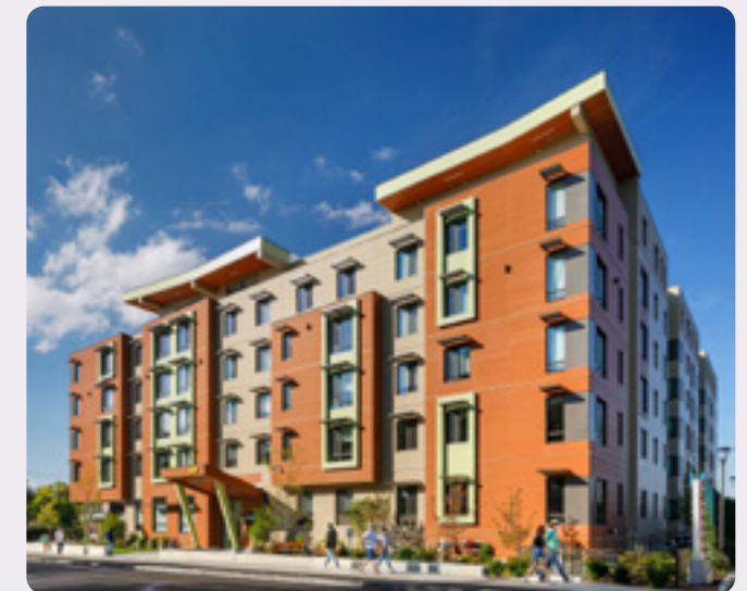
FIG. 83 Finch Cambridge uses heat exchange systems, highly insulative materials, and an airtight envelope, and earned a Passive House certification.
