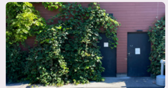
FIG. 87 Retail pavilion building in Cambridge Crossing incorporates greenery along the walls adjoining service doors.
