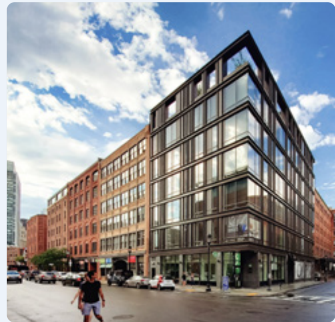
FIG. 7 Continuous streetwalls spatially define and frame Congress Street, Boston.
