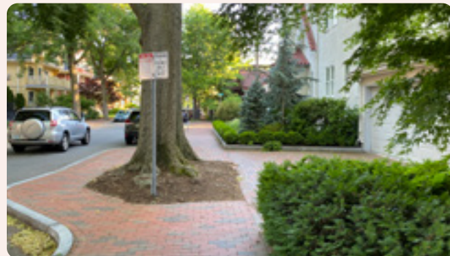
FIG. 185 Narrow residential sidewalk features a curb bump-out which allows for preservation of a large street tree, while providing adequate space for people walking and rolling.
