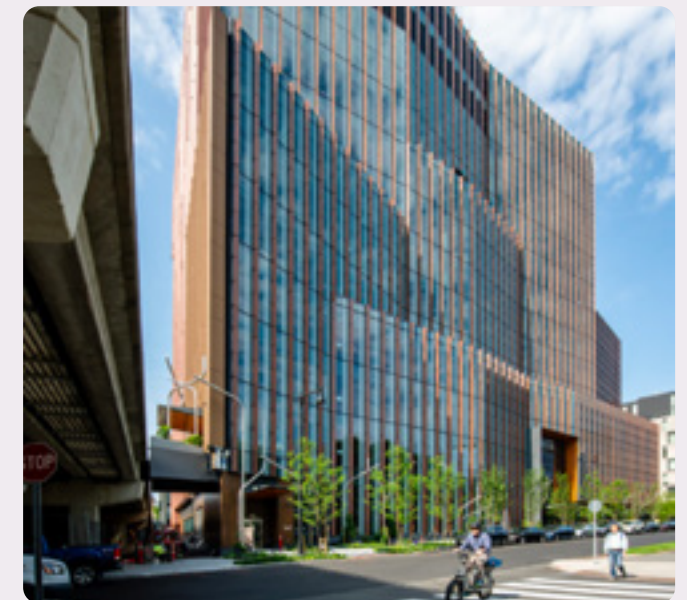
FIG. 81 The vertical fins on 411 Morgan Ave minimize glare and solar gain, while its orientation optimizes daylighting.
