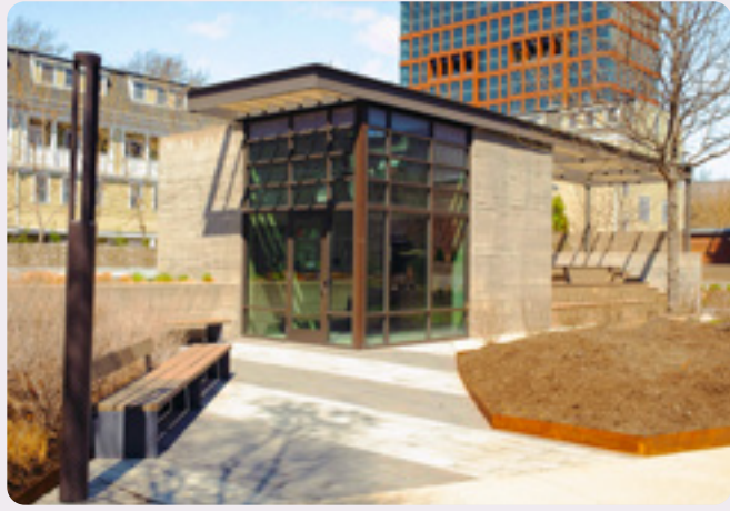
FIG. 100 A glass pavilion creates a dedicated pedestrian entrance to below grade parking, enhancing connectivity and promoting a more walkable, street-oriented environment
