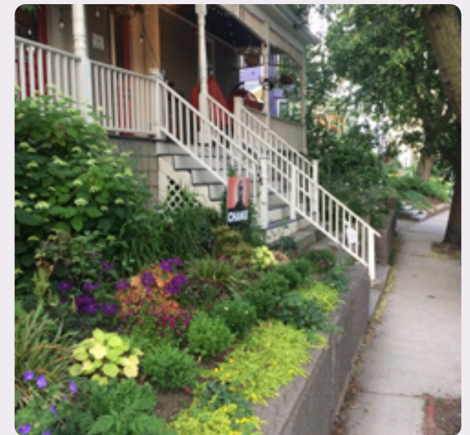
FIG. 55 Elevated residential ground floor in Somerville incorporates a low wall with planting and steps, rather than a sloped berm.
