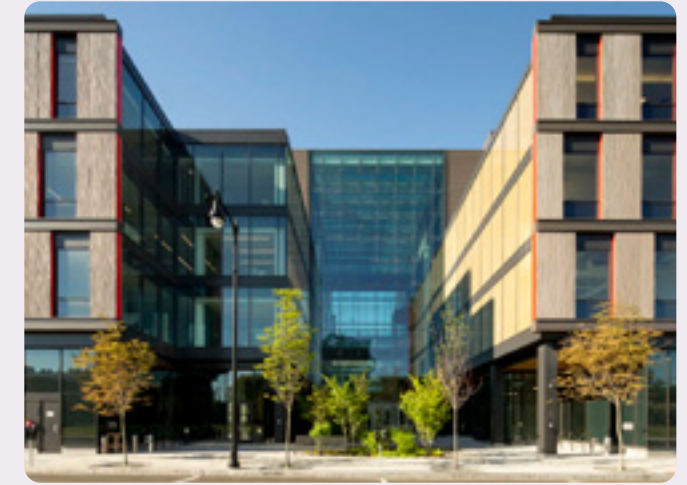
FIG. 37 A vertical break and forecourt is used to break down the length of this long building on Binney St.
