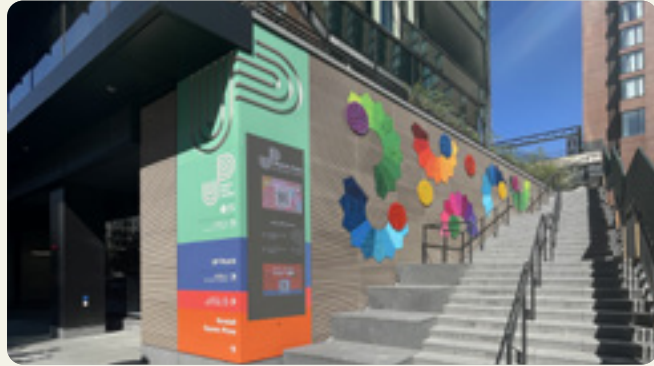
FIG. 149 Signage directs to a publicly-accessible rooftop garden.
