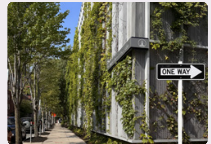
FIG. 99 Technology Square parking garage incorporates an attractive mesh screen and a green wall.
