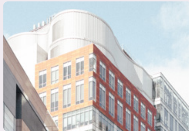
FIG. 88 Building on Ames St uses a curved wall to screen mechanical equipment, while adding visual interest to the building top.
