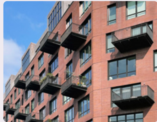
FIG. 73 Atelier 505 condominiums in Boston features balconies that create a rhythm along the building facade.
