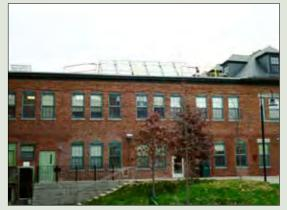
Six roof-mounted panels will heat domestic hot water for at the entire Blackstone site: the Steam Plant, the North office building and the LEED Platinum-certified South office building. This demonstration project is designed to evaluate the effectiveness of this renewable energy technology for potential applications across Harvard.
